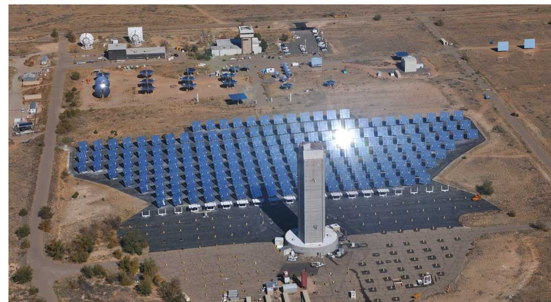
National Solar Thermal Test Facility at Sandia National Laboratories, Albuquerque, NM, with 200+ heliostats (~6 MW th )
