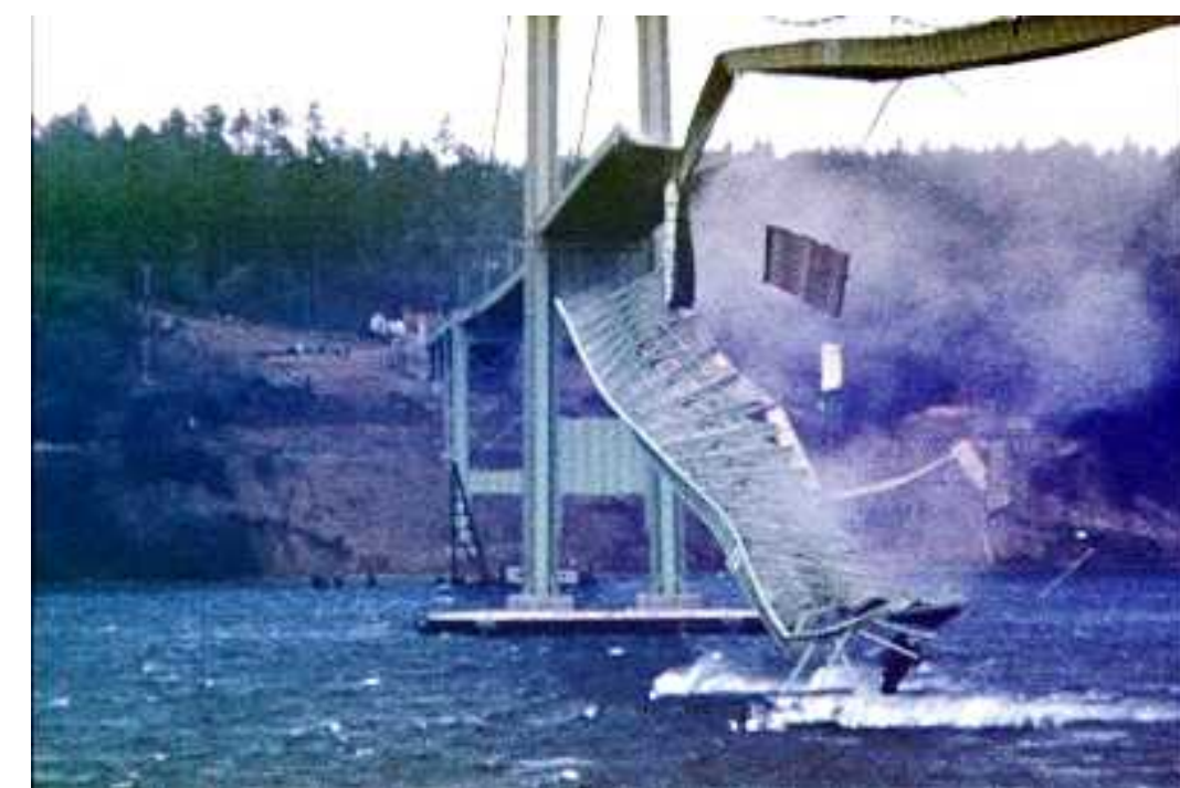
Tacoma Narrows Bridge collapsing under 40 mph winds (1940)
