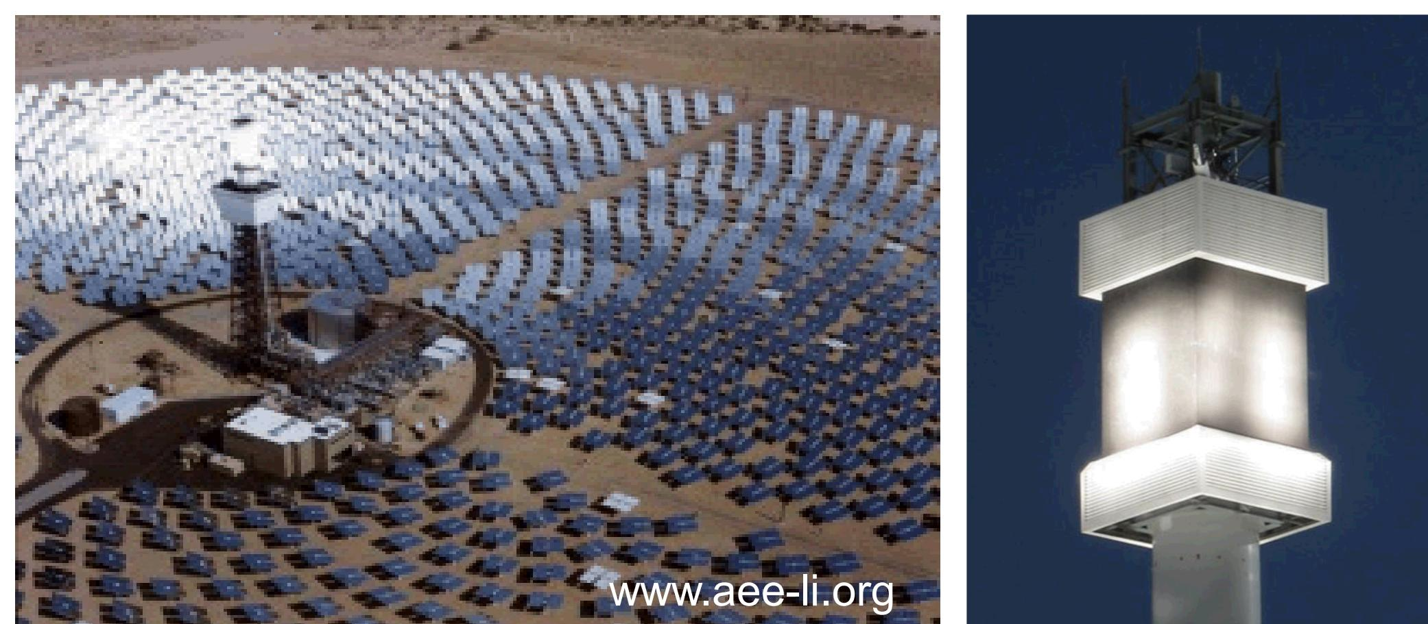
Concentrating solar power tower uses a field of mirrors (heliostats) to reflect the sunlight onto a central receiver. The energy absorbed is then used to heat a working fluid and in turn generate steam to power a turbine generator.
