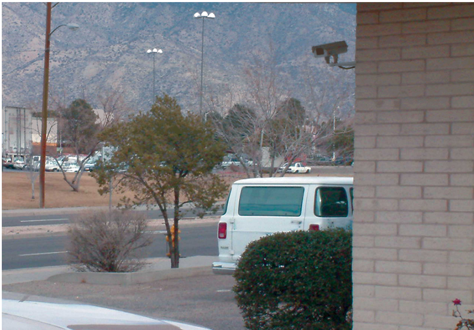
Figure 7.4 For most applications, a camera should be installed at a height of about 16 to 20 feet (while still capturing an effective view of the scene) to protect it from theft and vandalism. However, the design of the facility or the requirements of the scene to be captured may dictate a less-than-optimal installation location. The camera shown above was installed at a height of about 10 feet as the building is only one story and the cost of installing the camera on a pole would have been prohibitive for this center.
