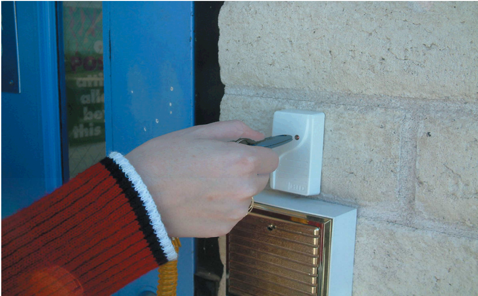
Figure 4.4 This is a key fob being held up to a proximity sensor. When the sensor validates the key fob, it will release the electronic door lock, thus allowing entry. Note the intercom box below the proximity sensor. This intercom allows visitors without a key fob to state their business and request entry. For this particular facility, the door intercom is answered by the office manager at an intercom unit on her desk. If the manager approves the visitor, she may simply press a release key on her intercom unit that will then release the electronic door lock for the authorized visitor.
