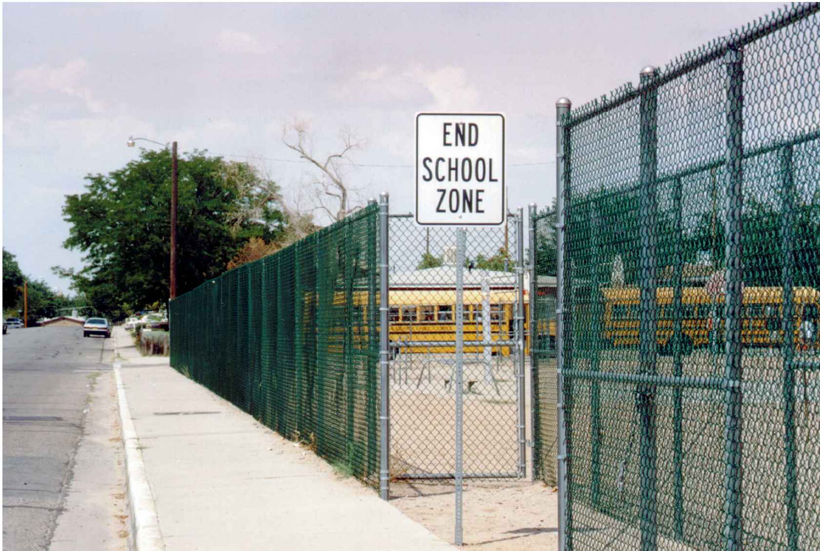
Figure 2.1 This 8-foot, smaller-mesh chainlink fence is around an elementary school. The school's problem with outside gang confrontations on the playground was completely eliminated after the fencing was installed.
