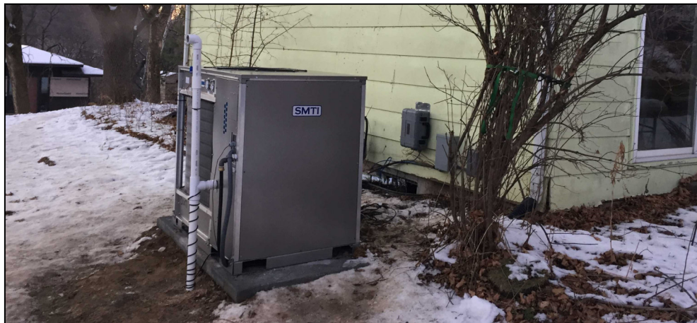
Figure 6: GAHP Prototype installed on Site 1 (Combi)
