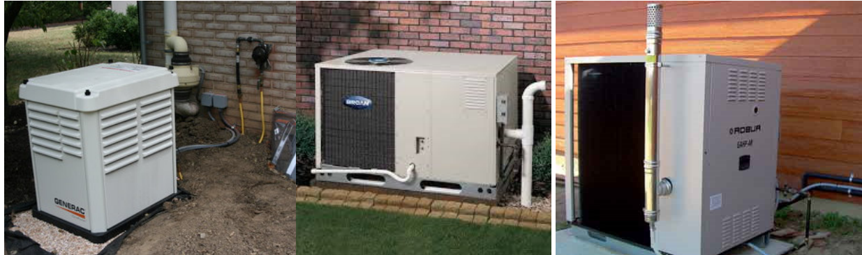
Figure C3: Residential Installations of Backup Generator (L), Gas Pack (C), and GAHP (R) [Source: Generac, Broan, Robur]
