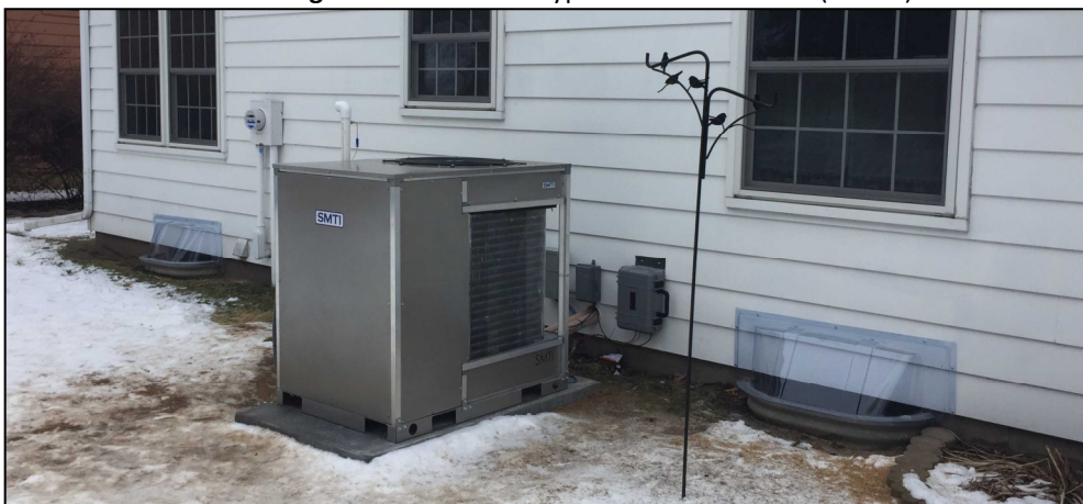
Figure 7: GAHP Prototype installed on Site 2 (Space heating only)
