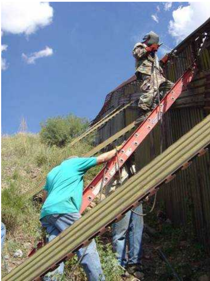
Installation of fiber optic sensor system on barrier wall in Nogales, AZ POE
