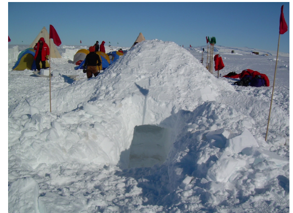
Close up the construction entrance, and open the real entrance (4-5 ft below grade)
