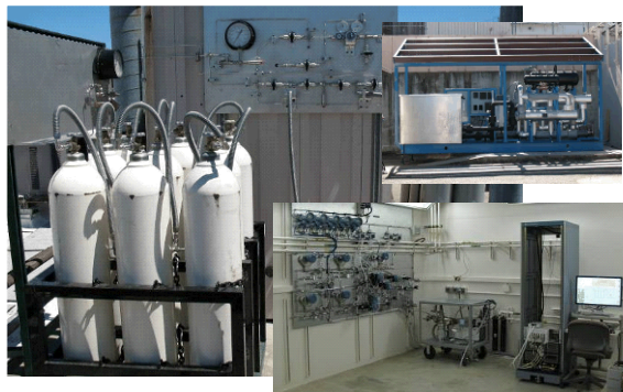
Figure 6 - High capacity, high rate, hydrogen fueling manifold
