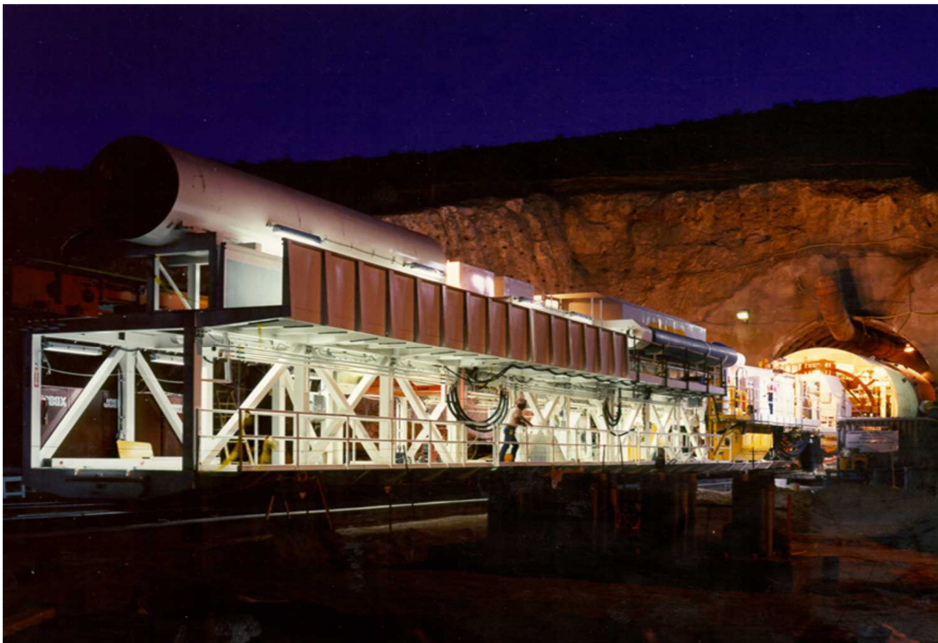
TWILIGHT VIEW OF THE 25 FT. TUNNEL BORING MACHINE ENTERING THE NORTH PORTAL
