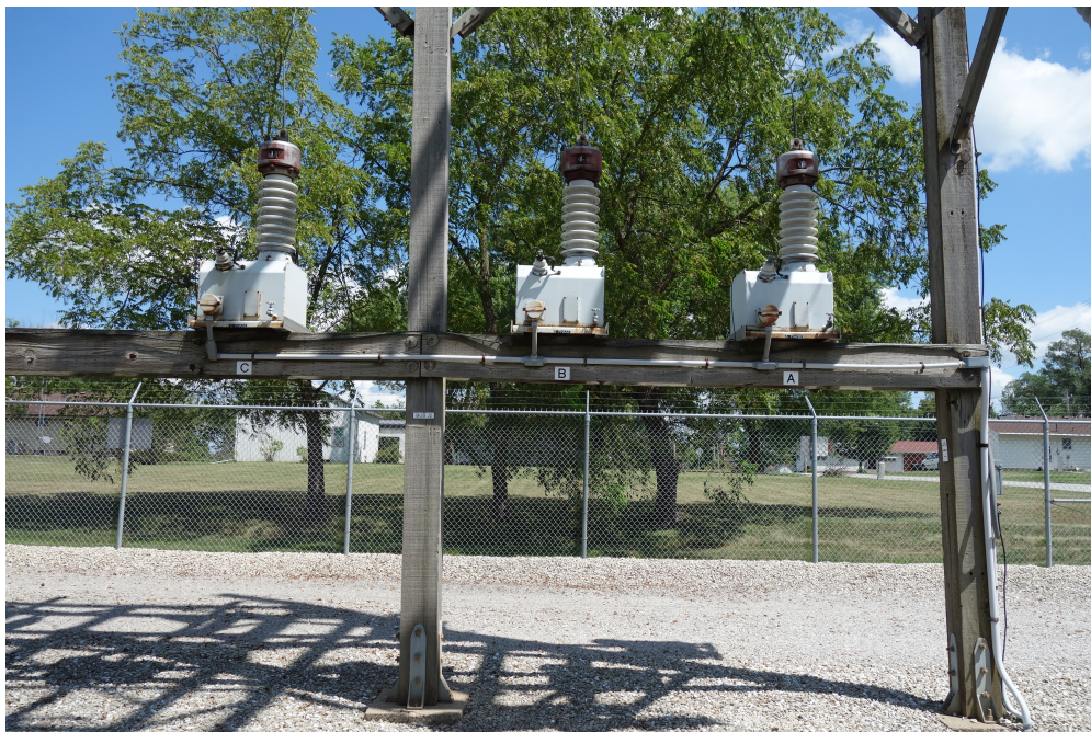
Figure 1.0.2. Instrument-to-trench elevated cables for substation Layout 2.
