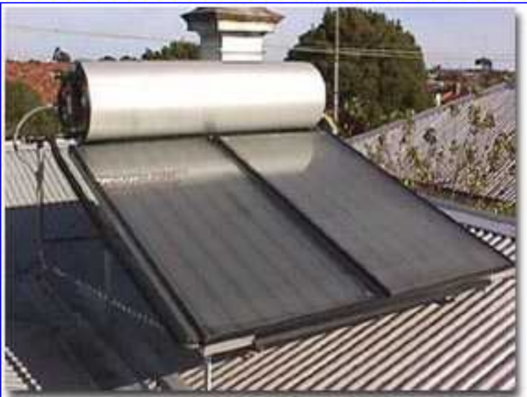
A solar water heater on a typical Australian suburban rooftop.
