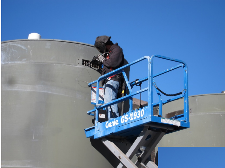
Removing the Gamma Shield
