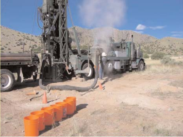
Collecting borehole cuttings from the drilling rig cyclone with a plastic bucket during the drilling of Borehole 58FF-GR-BH15. September 15, 2005. View to the northeast.
