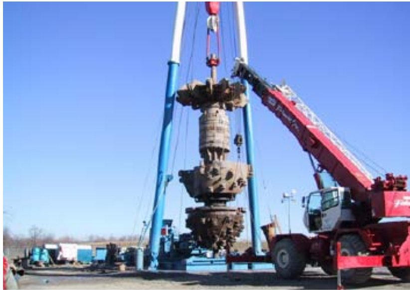
5.5 m Bottom Hole Assembly. Intake Air Shaft 100 m Deep – Kentucky, USA
