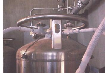
**Procedures** can also enhance safety, such as opening valves slowly to reduce the potential of flex line whipping and to minimize splashing and liquid boil-off, or properly venting pressure from transfer lines prior to cracking fittings.
