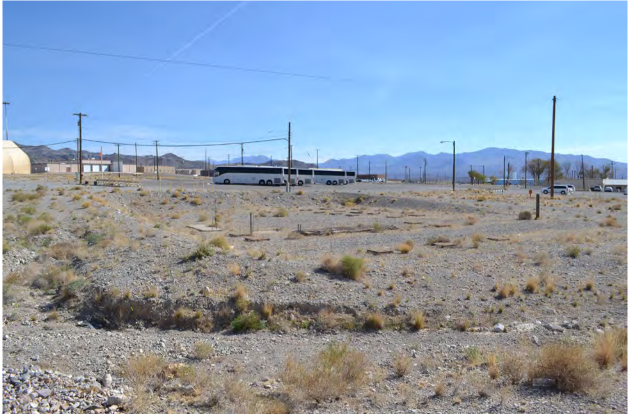
This photo, facing southeast, shows the remnants of the berm in the foreground that was built to guide stormwater around the substation (DRI 2017).
