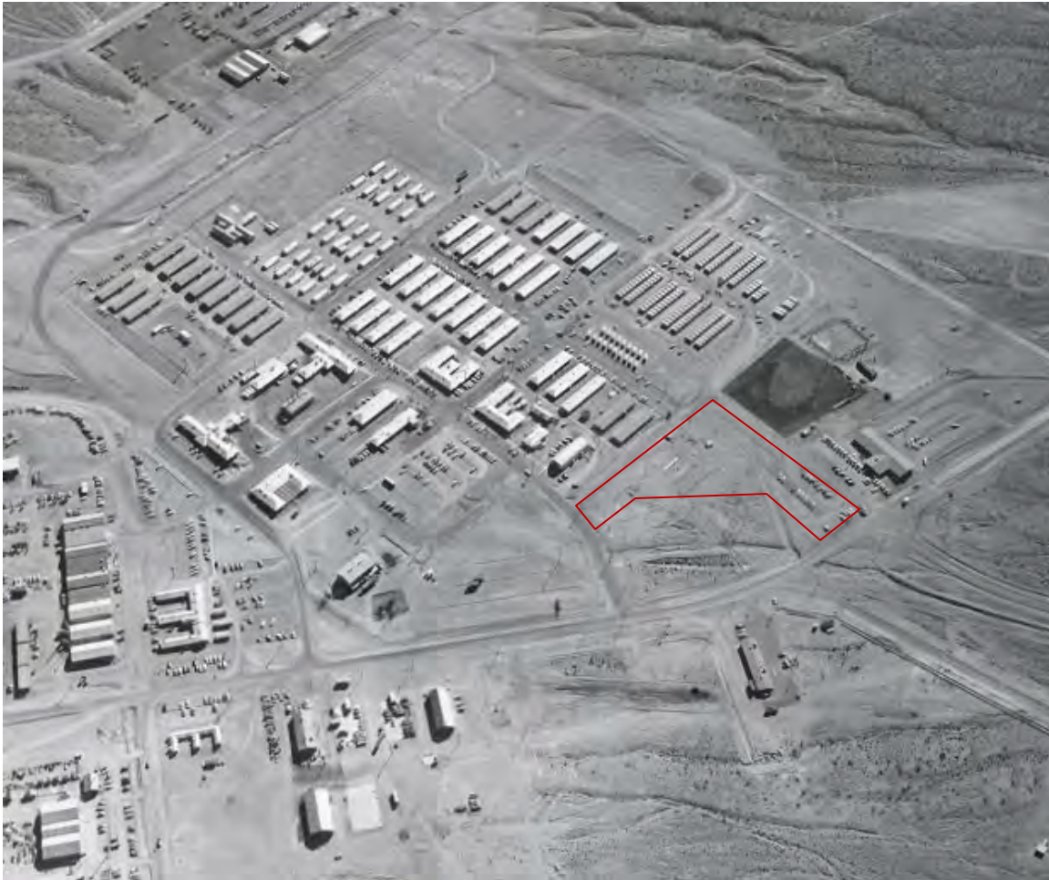
The general location of the future bus parking area (in red) in 1961 (REECO Photo 940-5, 1/24/1961, facing southeast).
