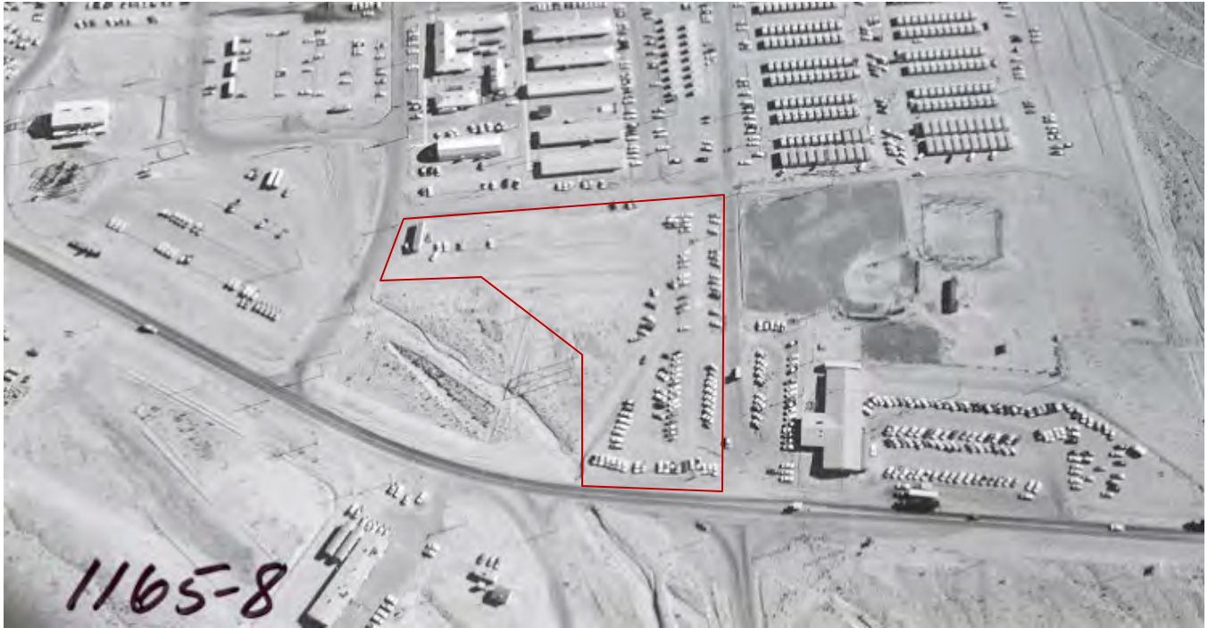
By late 1961, most of the area had been graded and partially paved (REECO Photo 1165-8, 12/7/1961, facing east).
