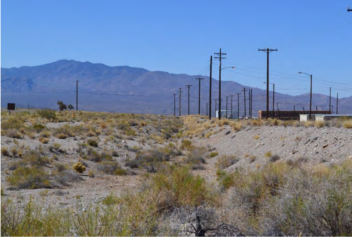
Drainage along the east side of Knothole Ave. Direction facing: South Photographer: Menocal
