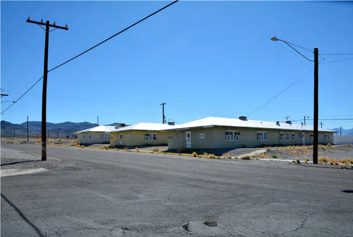
Ranger Ave. in front of Dorms B, C, and D between Snapper St. (in foreground) and Jangle St. Direction facing: East-southeast Photographer: DRI Date: 2015
