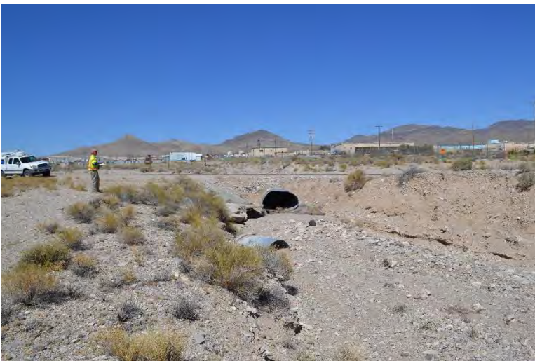
Culvert JF5. Direction facing: Northeast Photographer: Menocal Date: 2017
