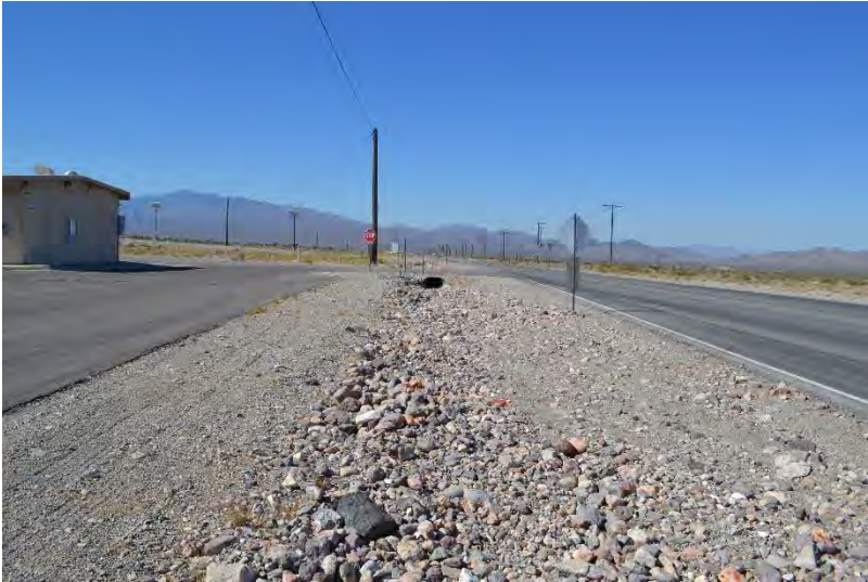
Culvert CM2. Direction facing: North Photographer: Menocal Date: 2017
