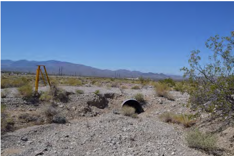
Inflow side of Culvert SA1. Direction facing: South Photographer: Menocal Date: 2017
