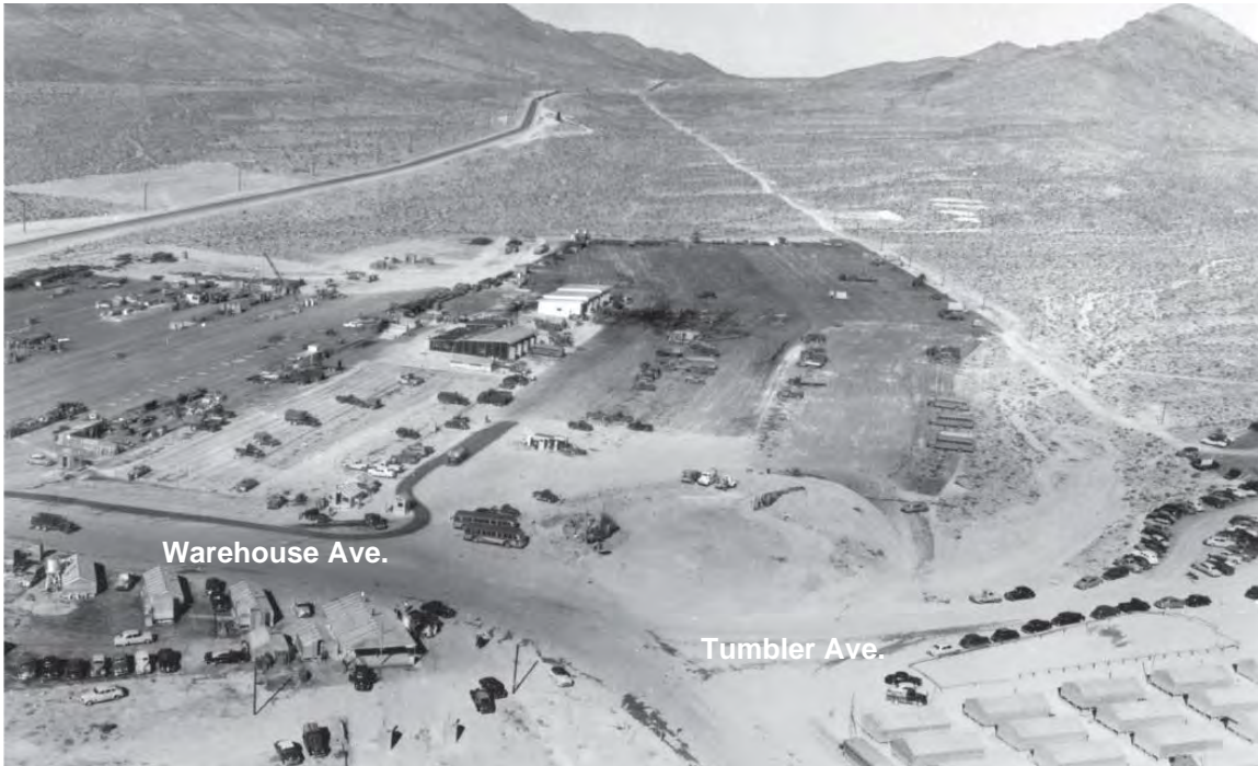
Roads that would become Warehouse Ave. and Tumbler Ave. during the early days of construction at Camp Mercury. Direction facing: Northeast Source: Fehner and Gosling 2006 Date: 1951
