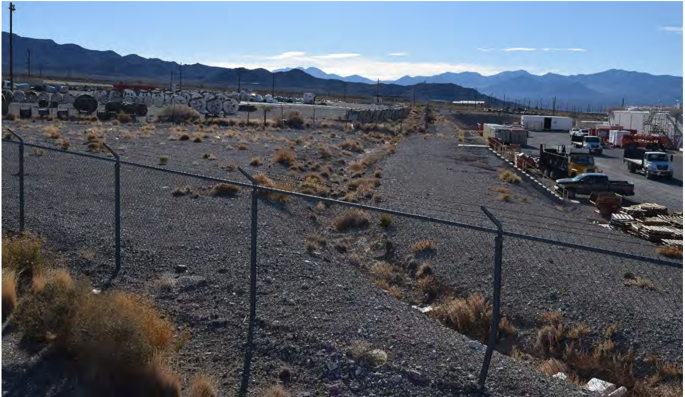
This ditch on the north side of Building 23-160 directs water around the building. The curve in the foreground feeds stormwater into the drainage along the east side of Mercury Highway. Elevation: N/A Direction facing: Southeast Photographer: DRI Date: 2018
