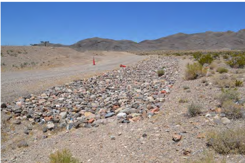
Riprap along NE edge. Direction facing: West-northwest
