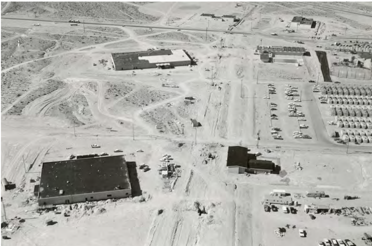
Trinity Ave. being reconstructed approximately 130 ft (40 m) to the south of its original location during a 1963 construction boom.
