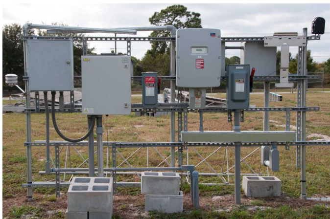
Representative inverter, disconnects, and monitoring equipment boxes at the FL RTC
