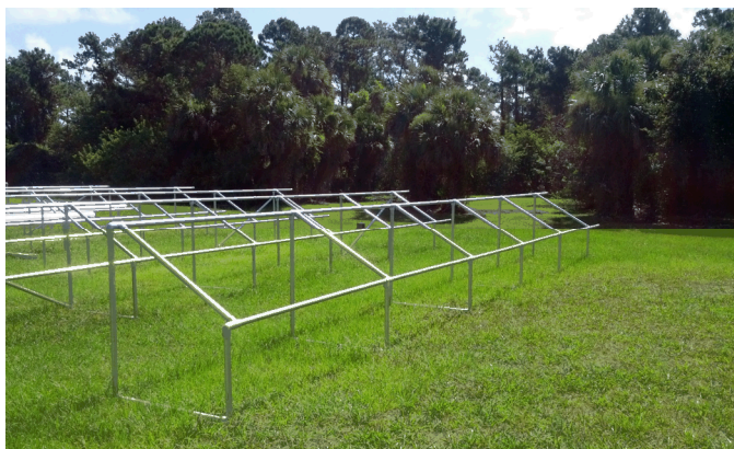
Racking being built for an RTC validation study
