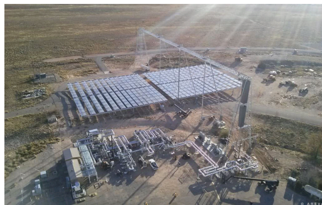
AREVA's molten salt energy storage demonstration plant installed at Sandia's National Solar Thermal Test Facility in Albuquerque, New Mexico.
