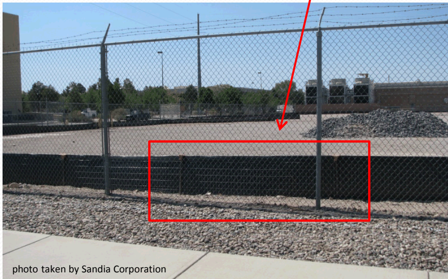
Silt Fence Perimeter Control
