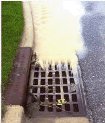
Chemicals allowed to discharge to storm inlet.
