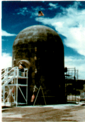
THE 1/6-SCALE REINFORCED CONCRETE MODEL
