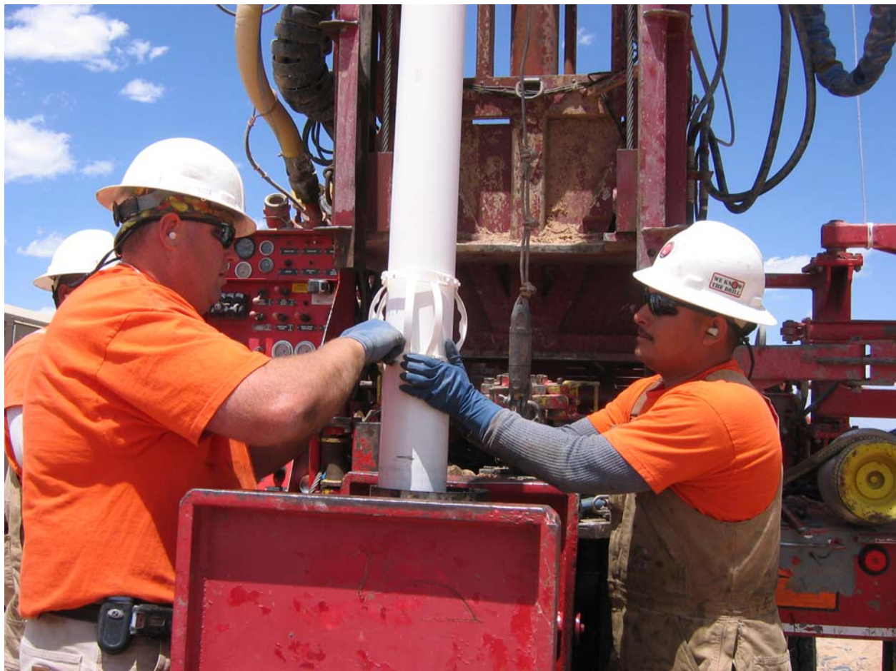
Figure 3-1 Installation of a Groundwater Monitoring Well with a PVC Centralizer
