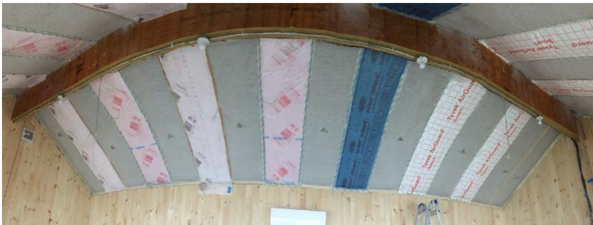
Figure 18. North-facing roof bays after vapor control membrane installation
