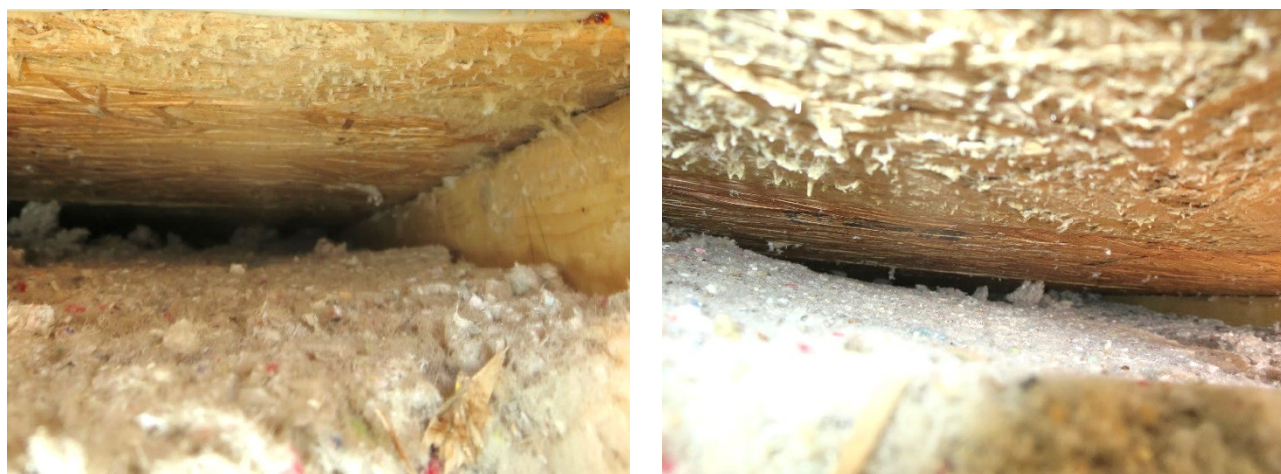
Figure 145. Settling of cellulose insulation on north-facing slope, Roof 5
