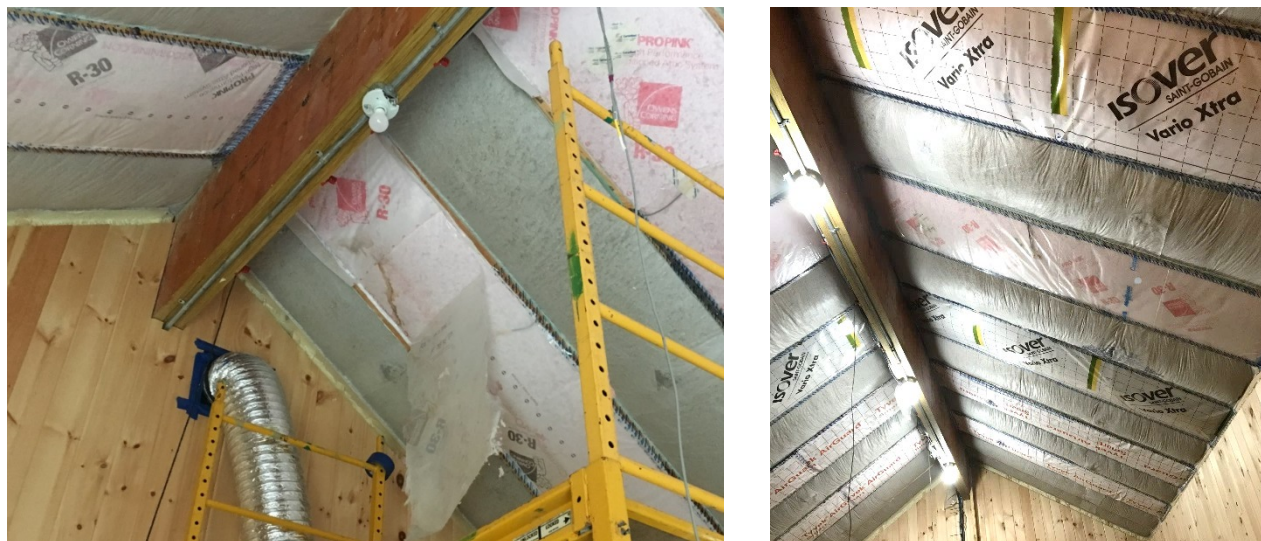
Figure 181. Removing old interior vapor control (left) and newly retrofitted bays (right)
