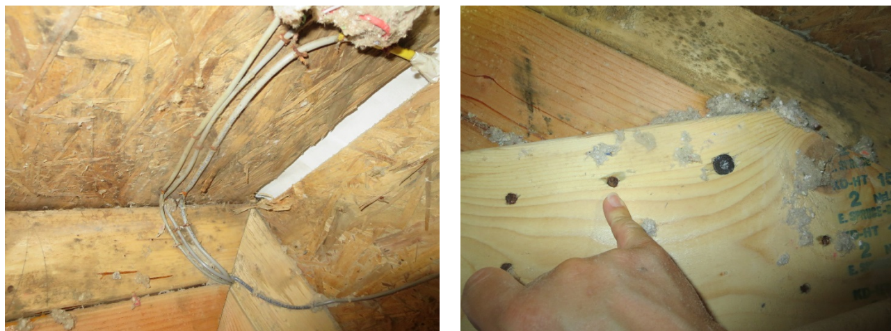
Figure 159. Roof 5 sheathing damage, east-side (left) collar tie rusted nails, rafter mold (right)
