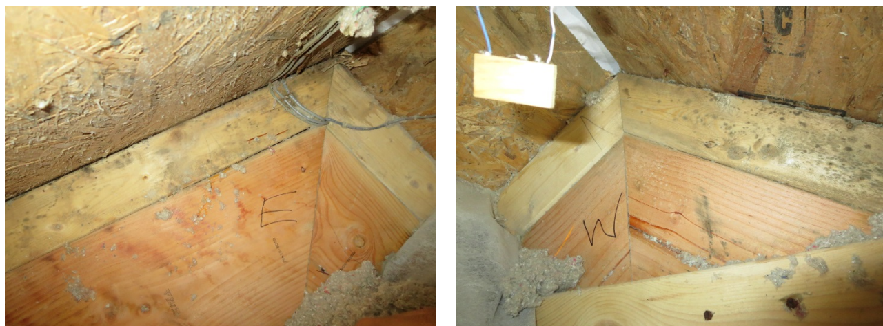
Figure 158. Roof 5 significant mold spotting on both east rafter (left) and west rafter (right)
