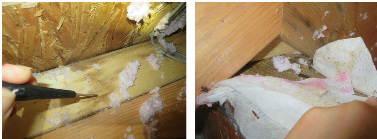
Figure 155. Roof 3 close-up of water staining on east rafter (left) ant infestation from adjacent bay (right)
