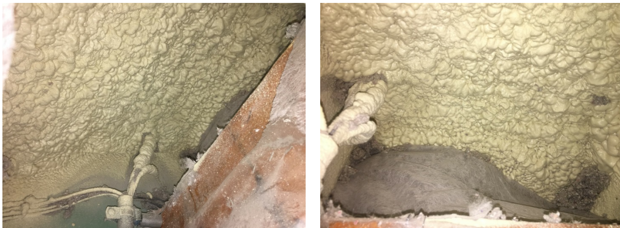
Figure 100. ccSPF surface conditions after removal of cellulose insulation
