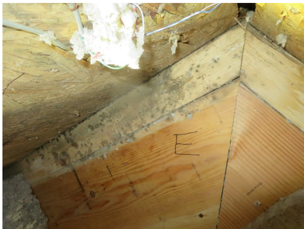
Figure 163. Roof 6 mold and staining on east rafter (left) and west rafter (right)
