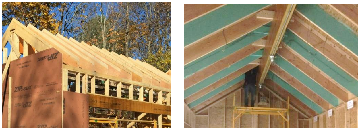
Figure 10. 2x12 and 2x4 rafters (left), air and vapor barrier on guard bay rafters (right)
