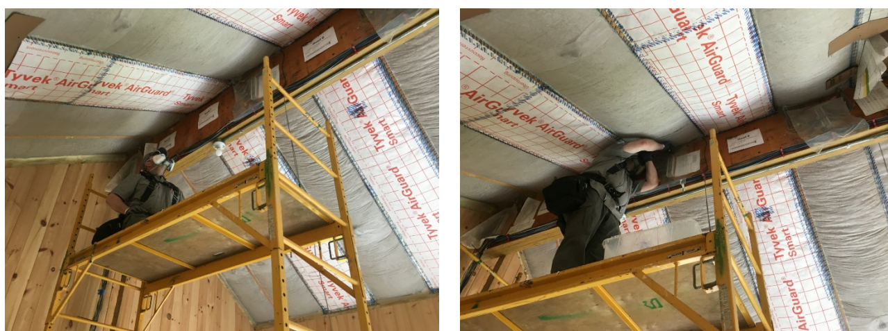
Figure 99. Cellulose insulation removal at guard bay between Roofs 6 and 7
