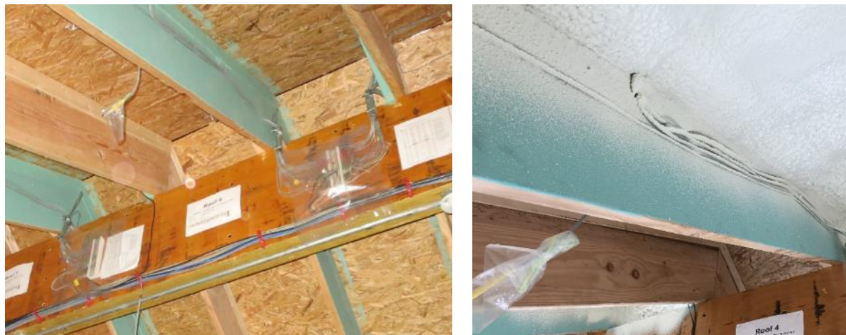
Figure 30. Conduit penetrations at guard bay (left), sealing of wiring holes with ccSPF (right)
