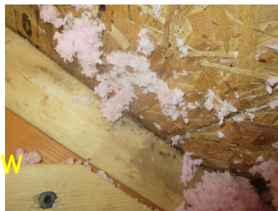
Figure 151. Roof 1 mold spotting on sheathing/framing (left) and bulk water stain on 2x4 (right)
