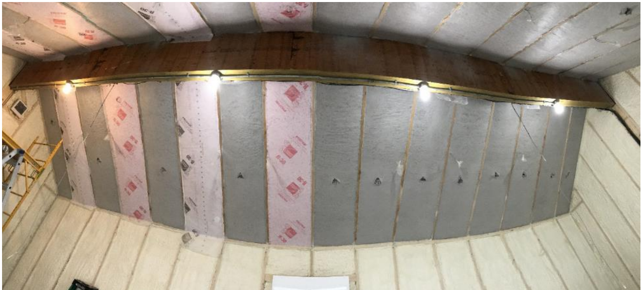
Figure 17. North-facing roof bays after netted fibrous insulation installation
