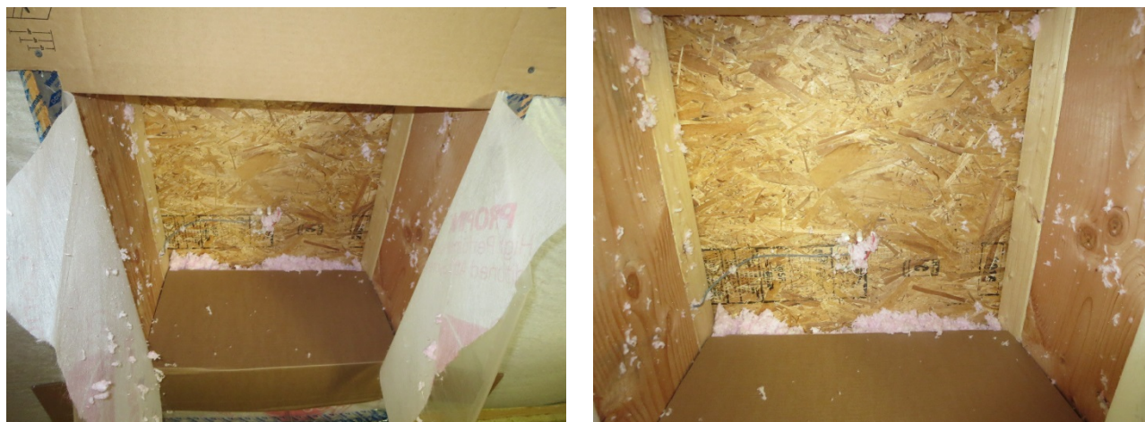
Figure 195. Opening at north-side roof sheathing and OSB conditions (Roof 2 fiberglass)
