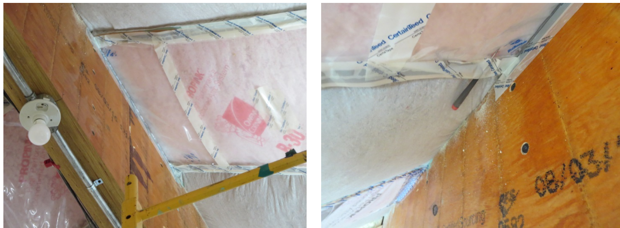
Figure 127. Roof 2, showing loss of adhesion of housewrap tape near ridge
