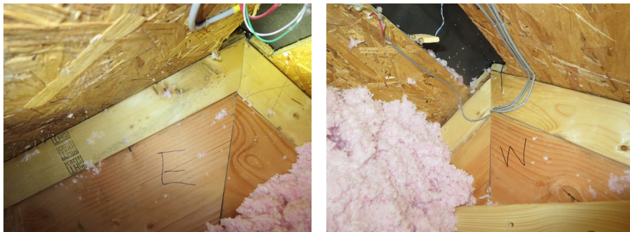
Figure 153. Roof 2 minor mold spotting on east rafter (left) clean conditions on west rafter (right)
