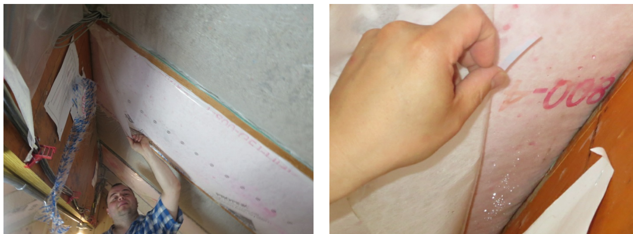
Figure 133. Roof 3 vapor retarder removal (left), condensation accumulation (right)
