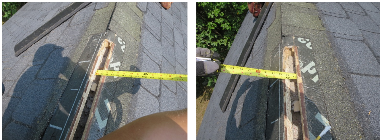
Figure 146. Settling of cellulose insulation on north (left) and south (right) slopes, Roof 6
