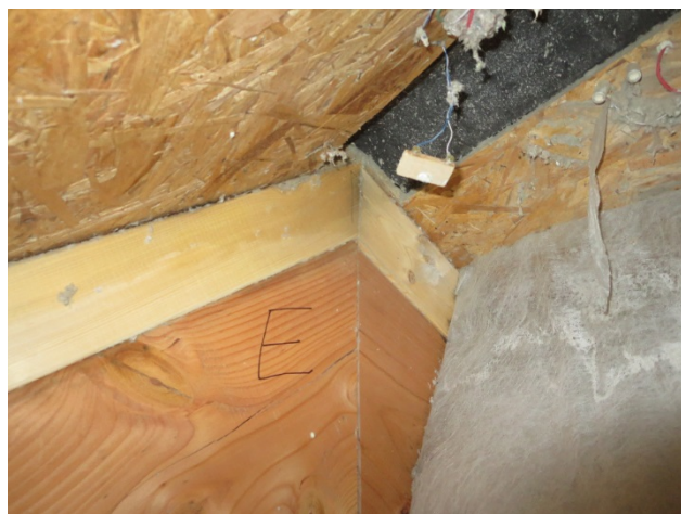
Figure 165. Roof 7 minimal damage to east rafter (left); mold and staining on west rafter (right)
