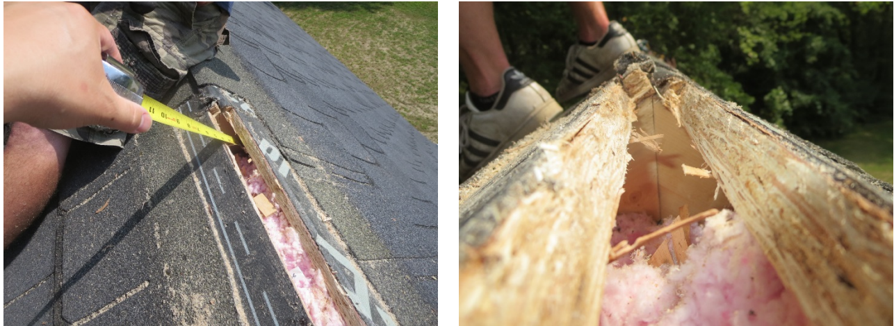
Figure 142. Settling of fiberglass insulation at ridge, Roof 4
