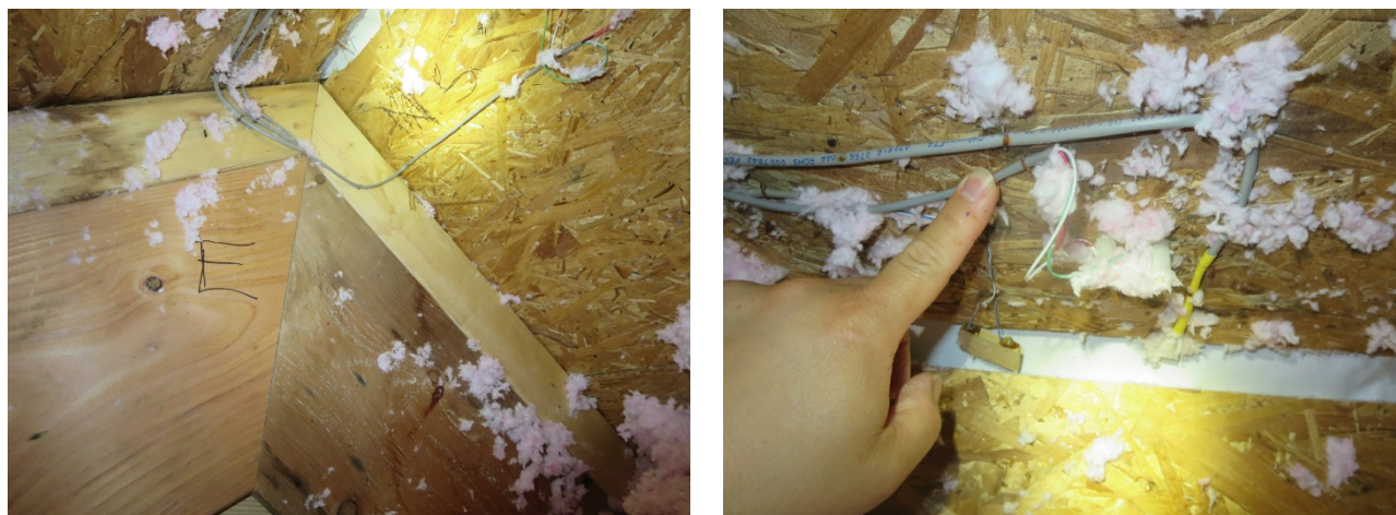
Figure 154. Roof 3 mold and staining on east rafter (left); sheathing damage and rusted staples (right)
