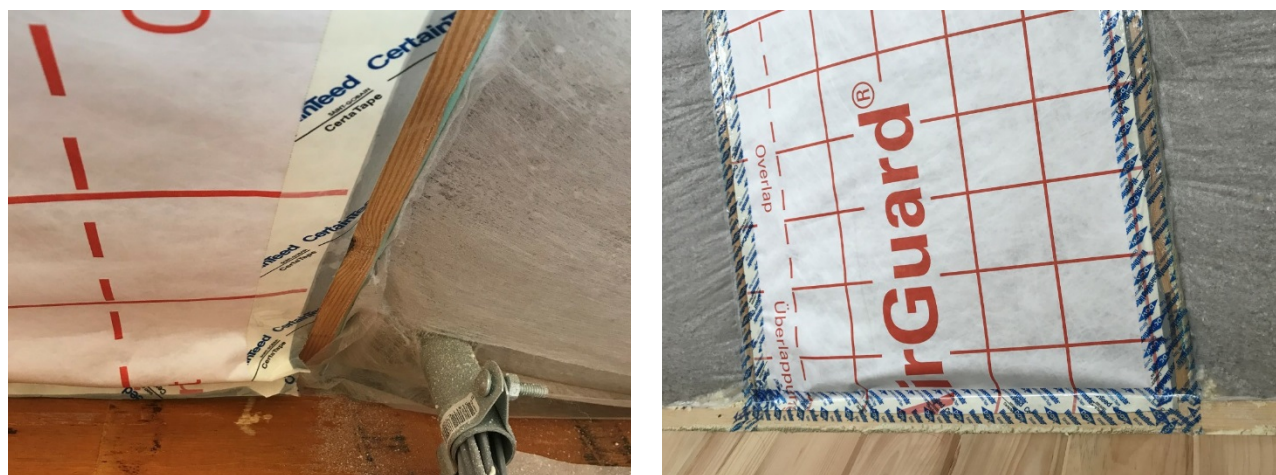
Figure 132. Cutting away failed housewrap tape (left) application of replacement tape (right)
