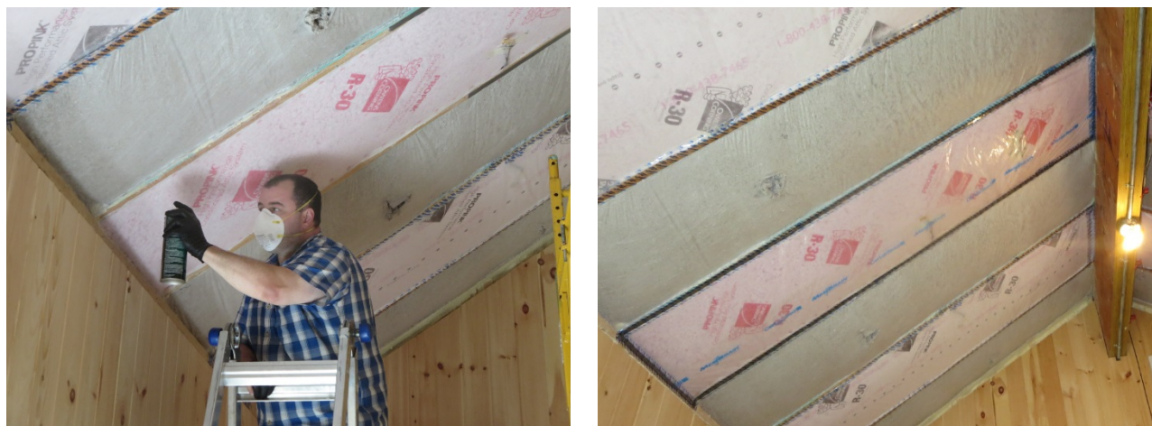
Figure 128. Reinstallation of Roof 2 vapor retarder: spray adhesive (left) and taped edges (right)
