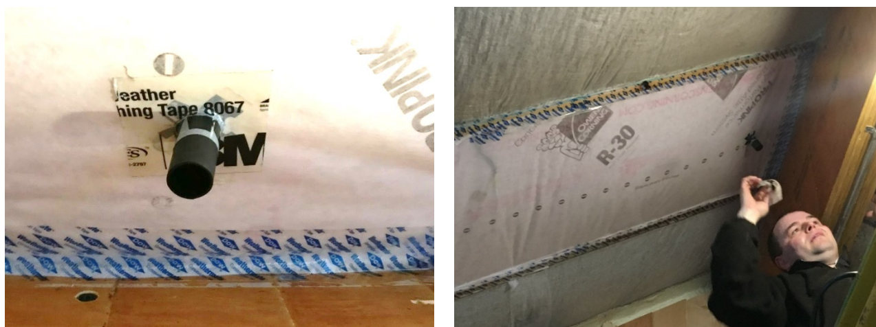
Figure 189. Roof ridge relief port close up (left); roof ridge relief port overview (right)
