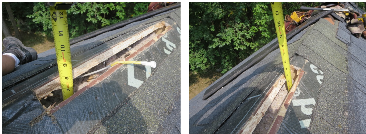
Figure 144. Settling of cellulose insulation at ridge, Roof 6
