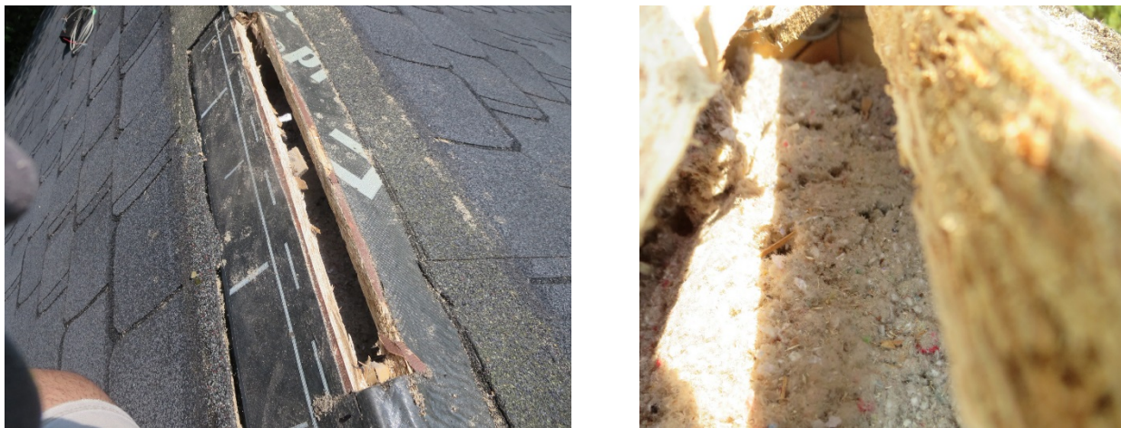
Figure 143. Settling of cellulose insulation at ridge, Roof 5
