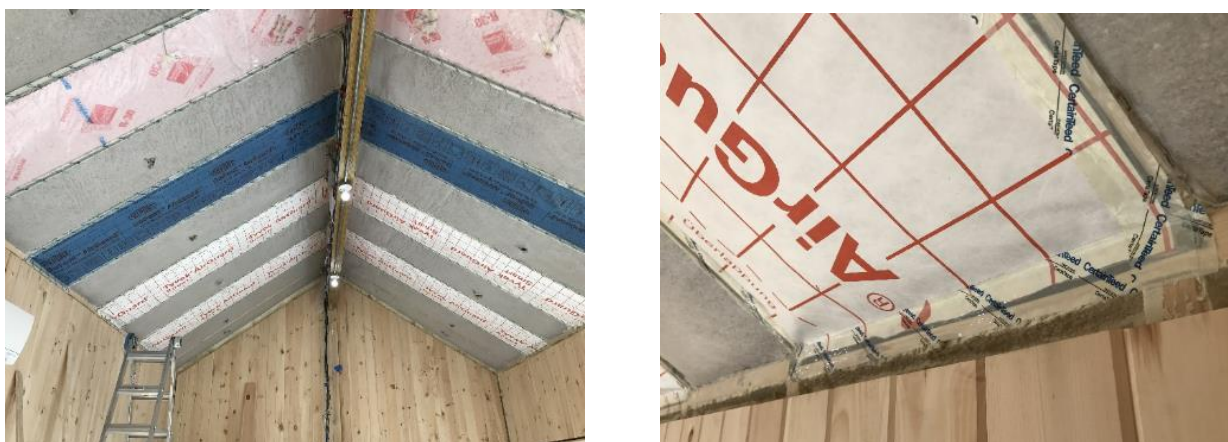
Figure 13. Interior vapor control membranes (left), double-tape air sealing detail (right)
