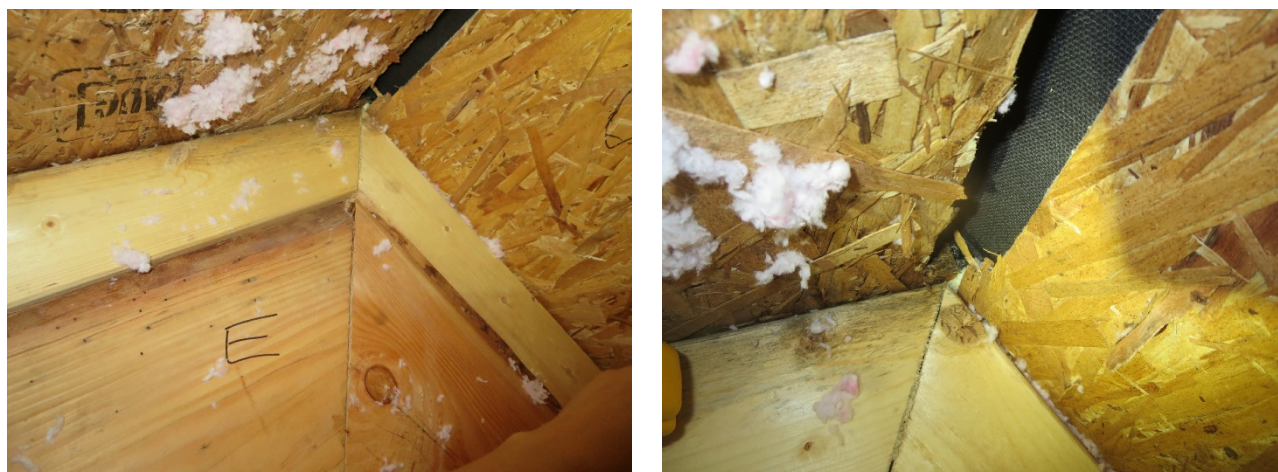
Figure 156. Roof 4 mold and staining on east rafter (left) close-up of east rafter and sheathing stains (right)
