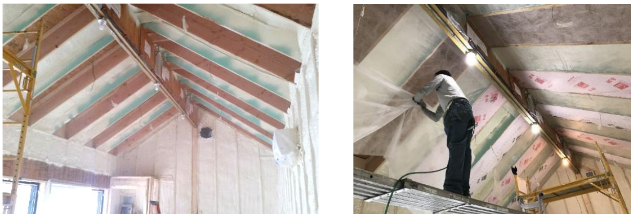
Figure 12. ccSPF insulation in guard bays (left); netting installation for blown insulation (right)
