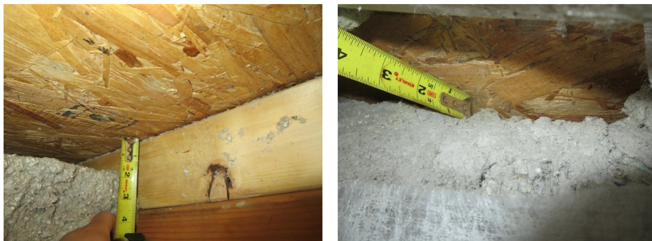
Figure 166. Roof 7 cellulose settling at north rafter bay (left) and south rafter bay (right)
