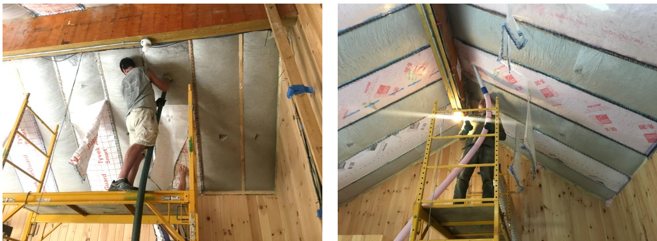
Figure 170. Reinsulation of roof ridge areas and repacking for cellulose (left) and fiberglass (right)
