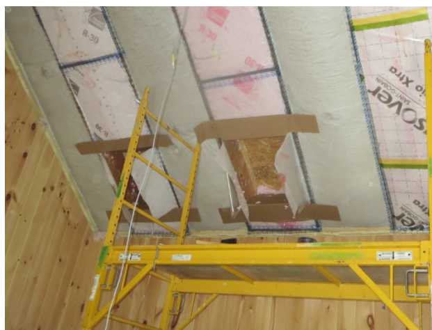
Figure 193. Installation of cardboard baffles for north roof sheathing examination
