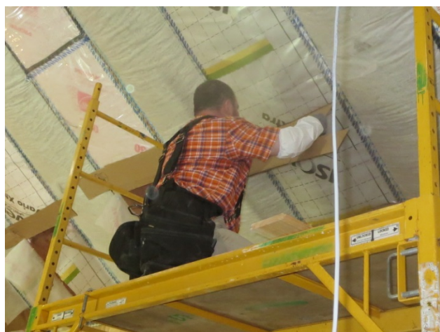
Figure 193. Installation of cardboard baffles for north roof sheathing examination
