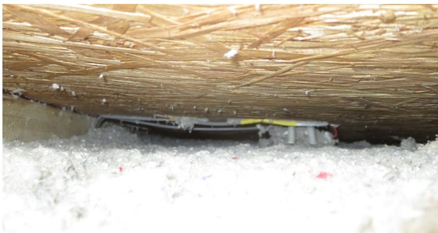
Figure 164. Roof 6 cellulose settling and gap at north rafter bay; note cellulose stuck in instruments
