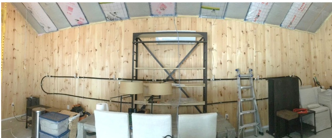
Figure 186. Overview of air injection system, showing manifold loop
