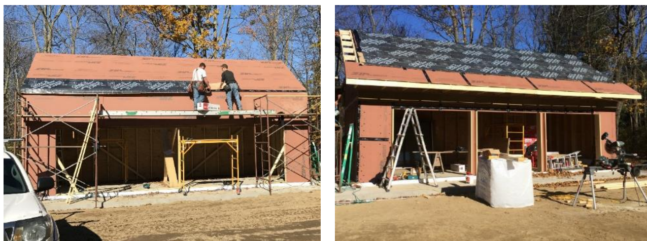
Figure 9. Roof-to-wall air barrier connection (left), eaves and rakes attached (right)
