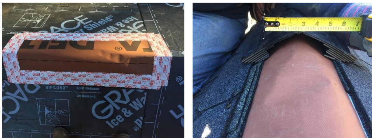
Figure 22. Diffusion vent ridge detail, showing taped membrane (left) and ridge vent cap (right)
