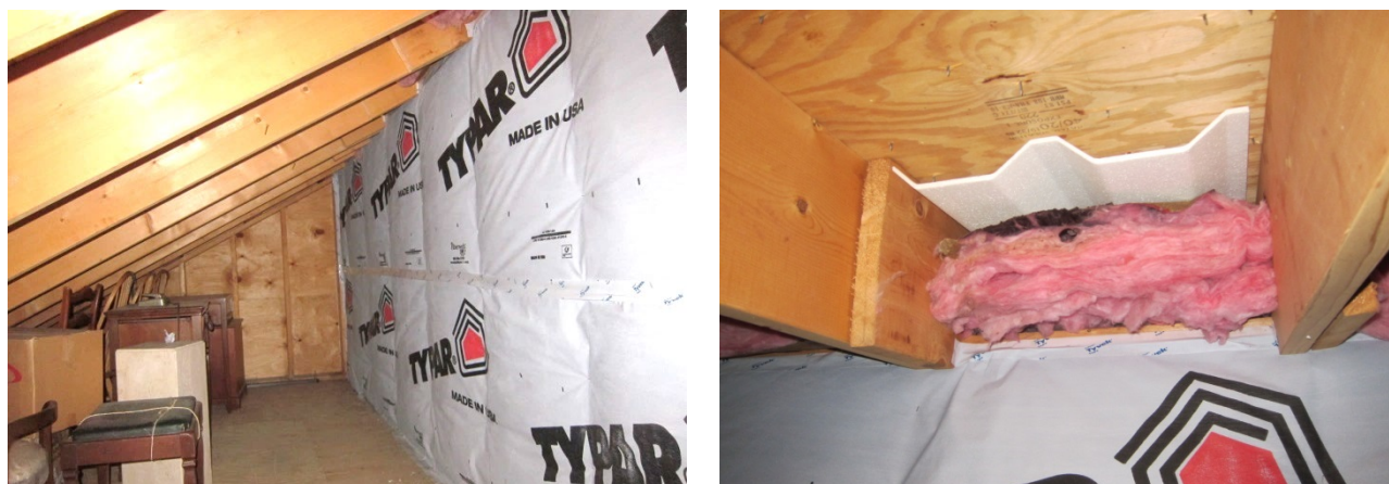
Figure 105. Attic kneewall area (left) with polystyrene vent chute over fiberglass batt insulation (right)
