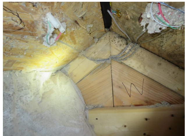
Figure 163. Roof 6 mold and staining on east rafter (left) and west rafter (right)
