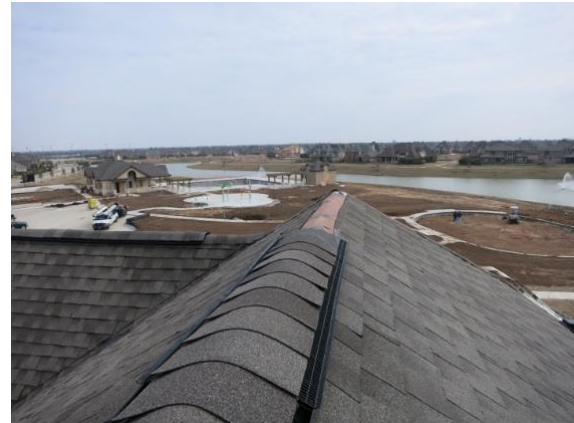
Figure 3. Houston diffusion vent showing ridge condition
