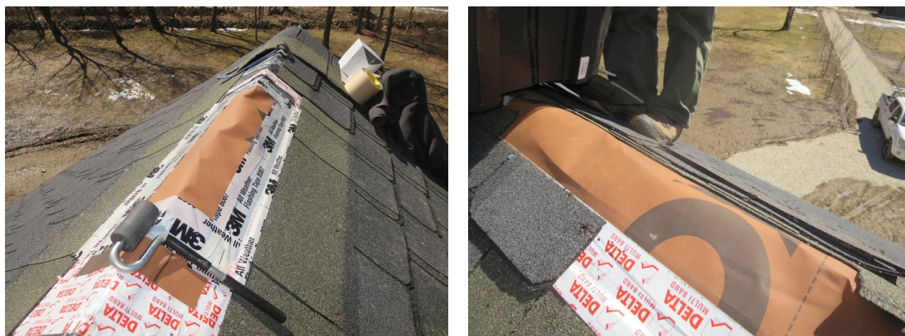
Figure 123. Reassembled Roof 1 diffusion vent (left) and Roof 2 examination (right)
