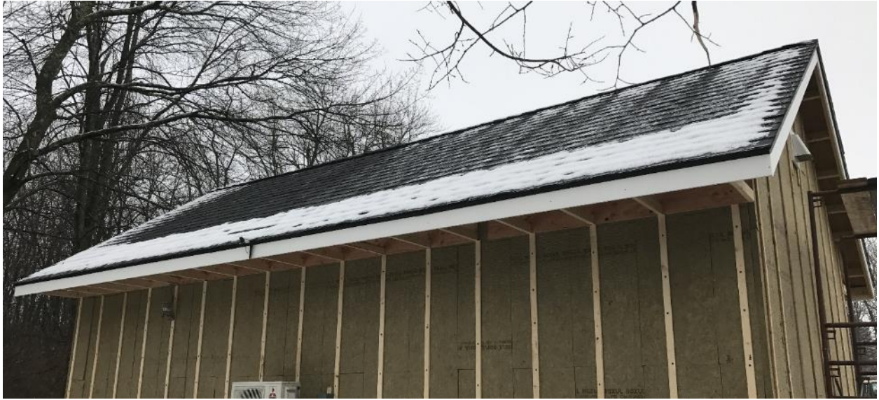
Figure 109. Snow melt patterns on north-facing roof, showing rafter thermal bridging
