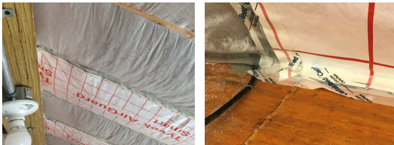
Figure 131. Tape adhesion loss at Roof 6 along rafter and at ridge
