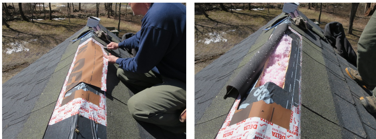
Figure 121. Cutting open existing diffusion vent ridge membrane, after vent removal
