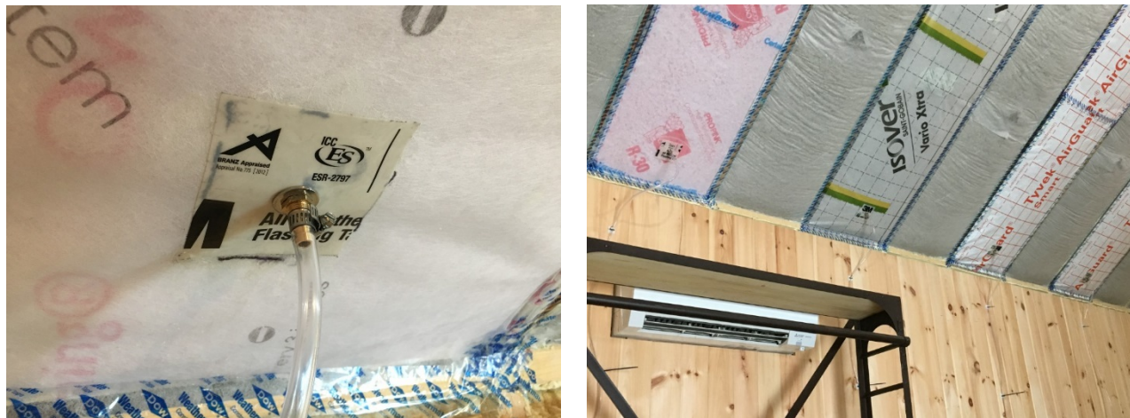
Figure 188. Tubing hose barb penetration (left); tubing attachment for Roofs 4–7 (right)
