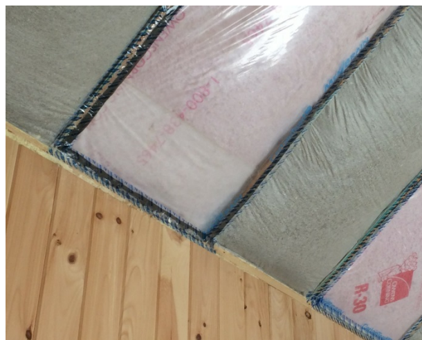
Figure 130. Roof 3 north vapor retarder failure (January)
