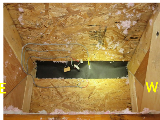
Figure 152. Roof 1 ridge sheathing conditions (left) and east-side rafter (right)
