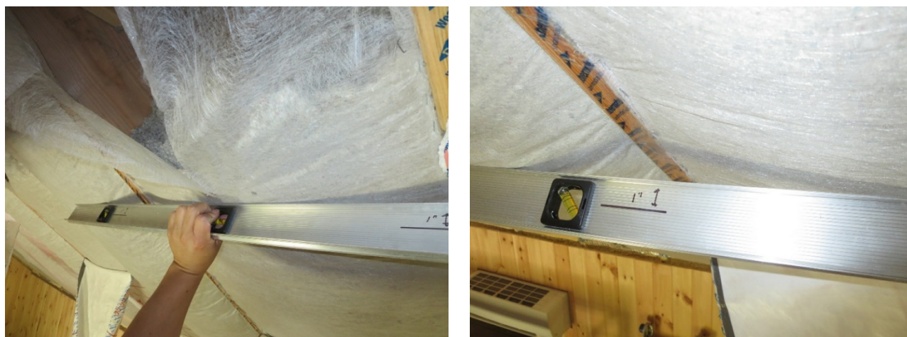
Figure 161. Cellulose netting belly (left); belly depth ~1 to 1.5 in. (right)
