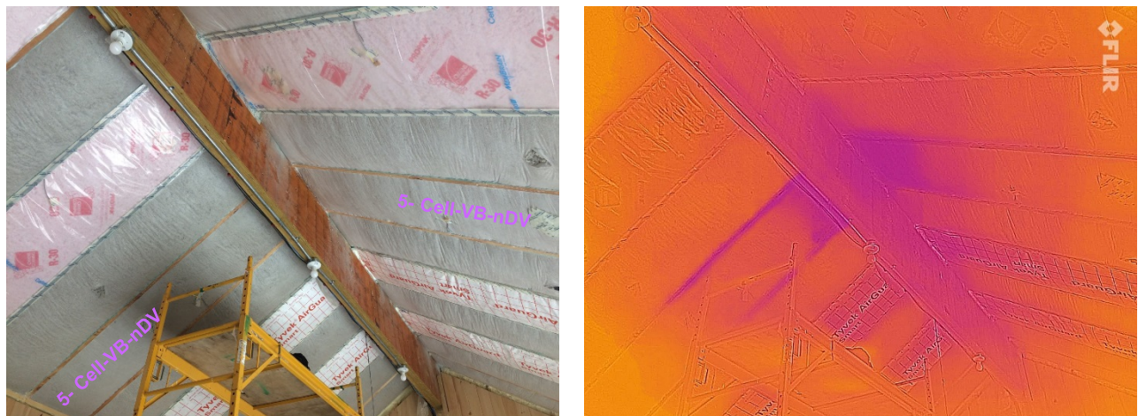
Figure 138. Visual and infrared image of Roof 5 (cellulose) after fixed-perm vapor retarder removal
