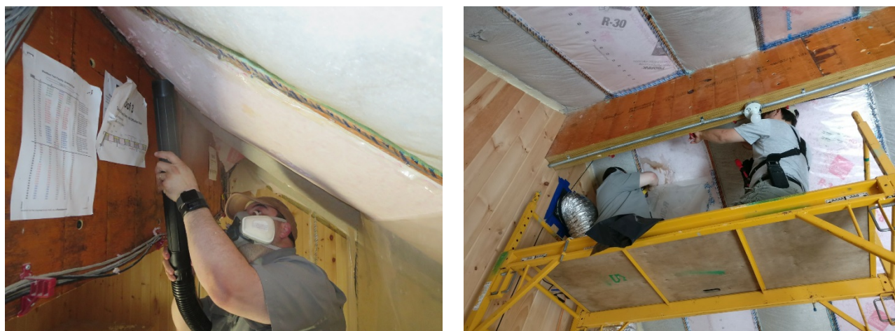
Figure 148. Removal of fiberglass insulation at ridge of Roof 1
