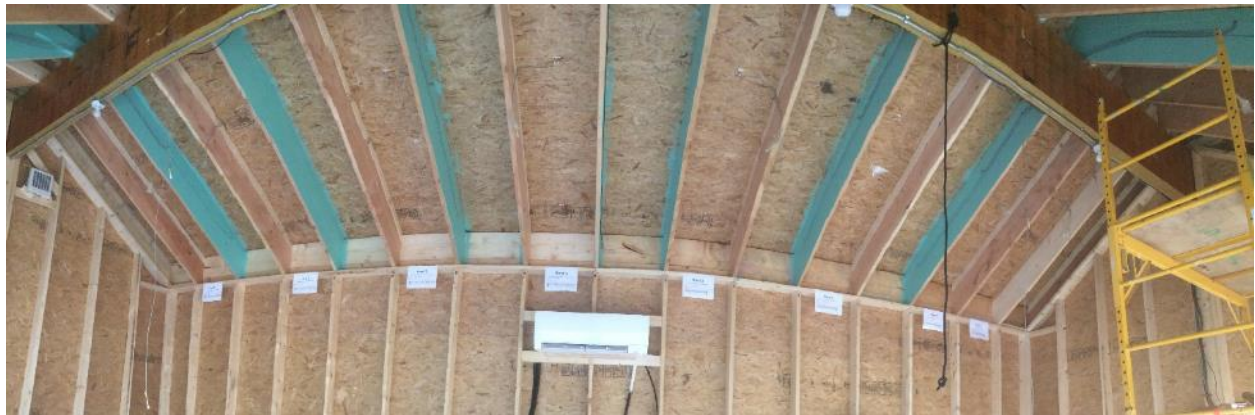
Figure 15. North-facing roof bays after instrumentation
