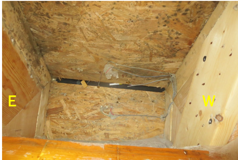
Figure 162. Roof 6 peak overview; extensive mold on east rafter and north sheathing
