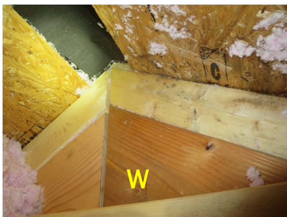
Figure 151. Roof 1 mold spotting on sheathing/framing (left) and bulk water stain on 2x4 (right)
