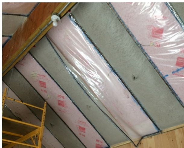
Figure 129. Roof 3 north vapor retarder failure (October)
