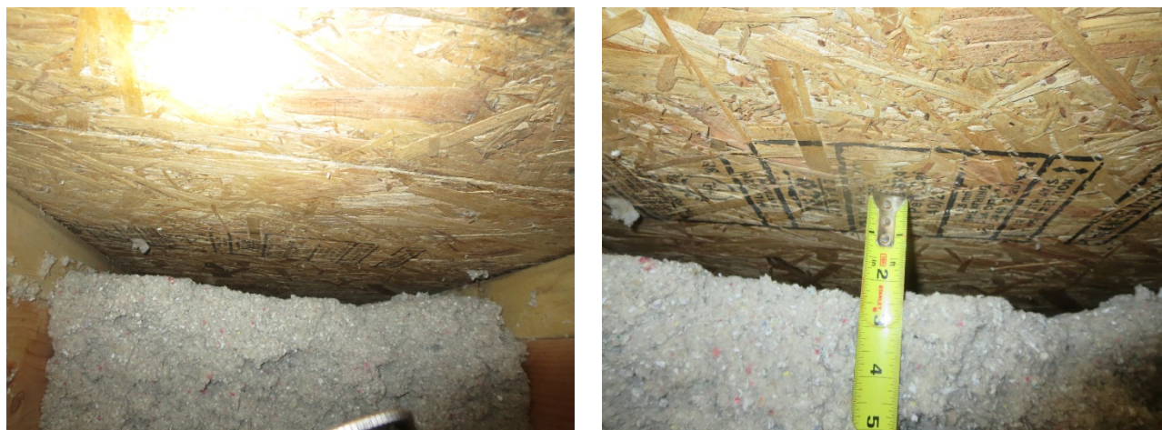
Figure 160. Roof 5 north-side cellulose settling (left); gap size 2 to 2.5 in. (right)
