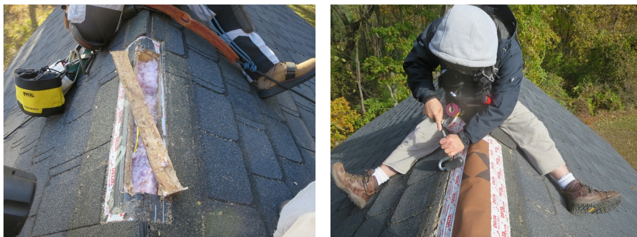
Figure 178. Retrofitting diffusion vent opening (left) and taping (~25-perm) diffusion vent (right)
