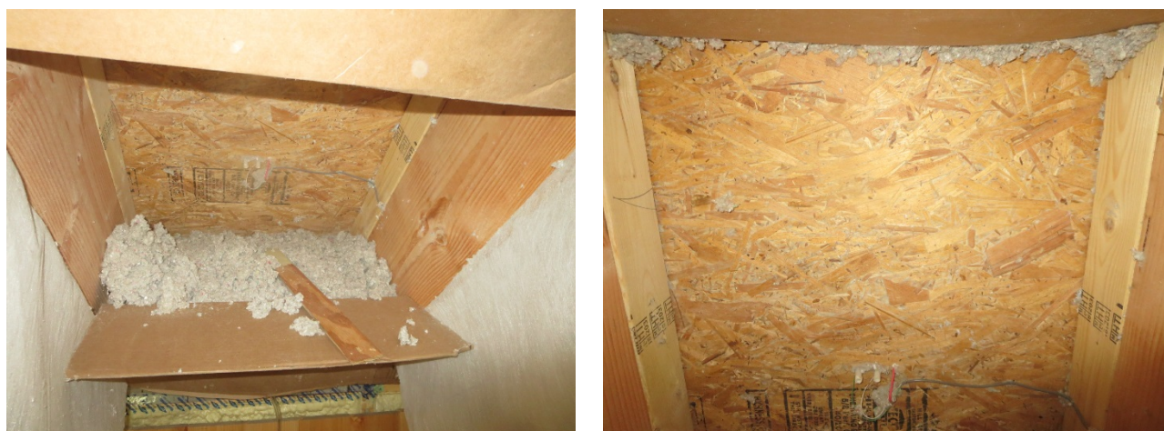
Figure 196. Opening at north-side roof sheathing and OSB conditions (Roof 5 cellulose)
