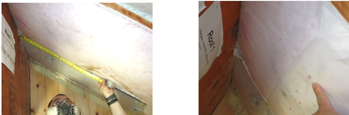
Figure 150. Roof 1 water staining on netting (left) and pink spotting on fixed-perm vapor barrier (right)
