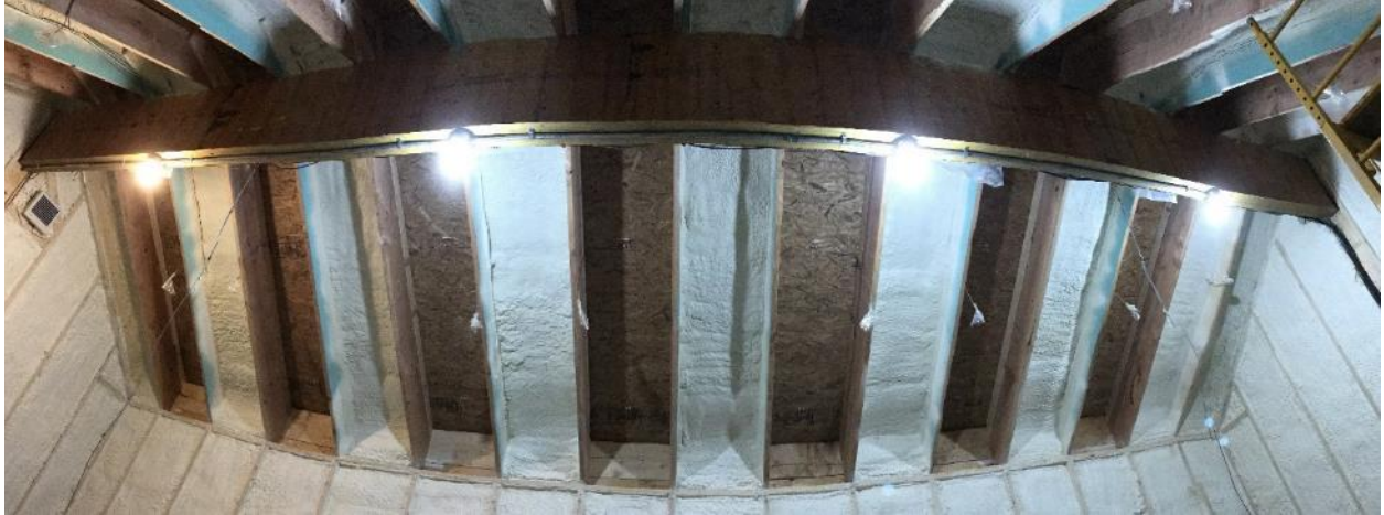
Figure 16. North-facing roof bays after spray foam installation
