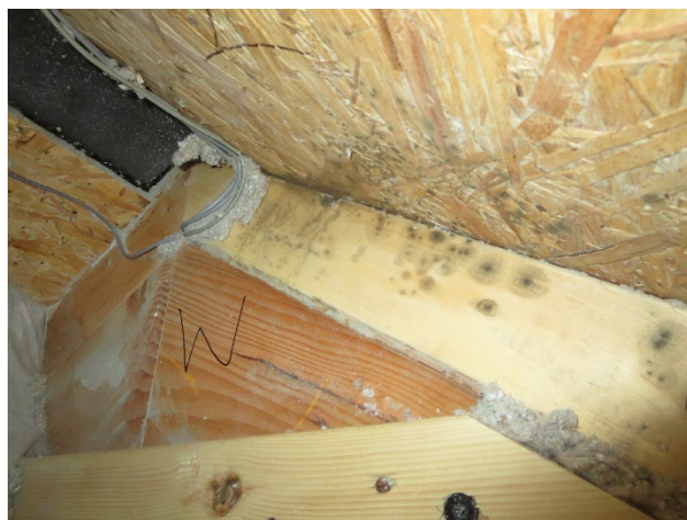
Figure 165. Roof 7 minimal damage to east rafter (left); mold and staining on west rafter (right)
