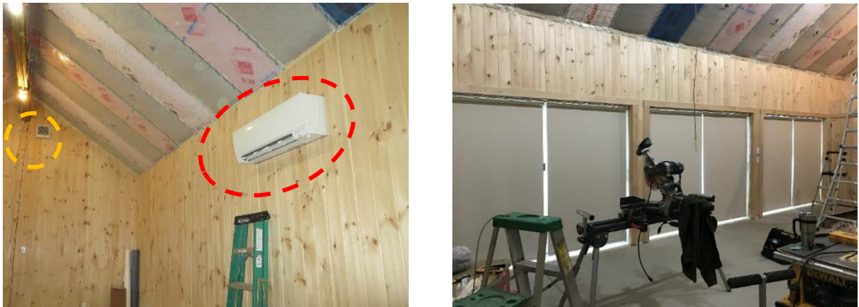
Figure 14. Mechanical systems (left) and solar control shades (right)
