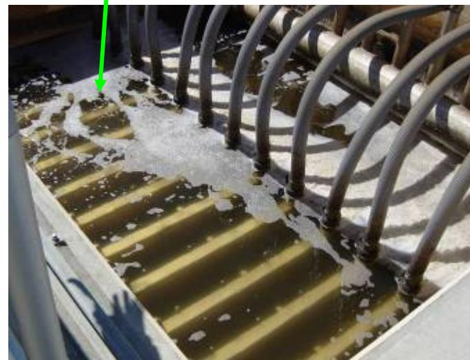
**Submerged microfiltration for treated wastewater effluent**
