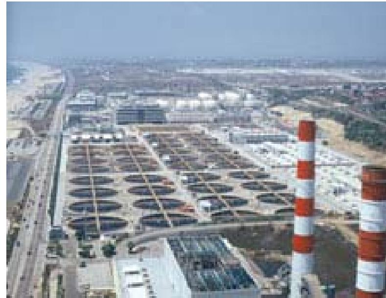
**10% of discharge from this plant is sent to microfiltration plant to purify for groundwater injection**
