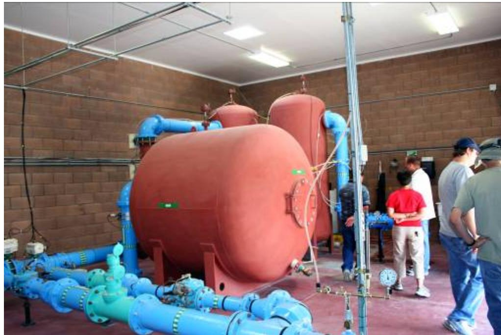
**Iron and manganese often occur together in groundwater and can also be removed together in a precipitation filtration reactor**
