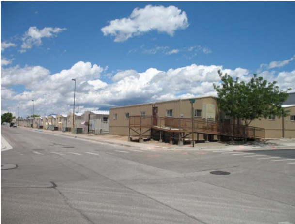
14 th St. & L Ave. Area– NE View
