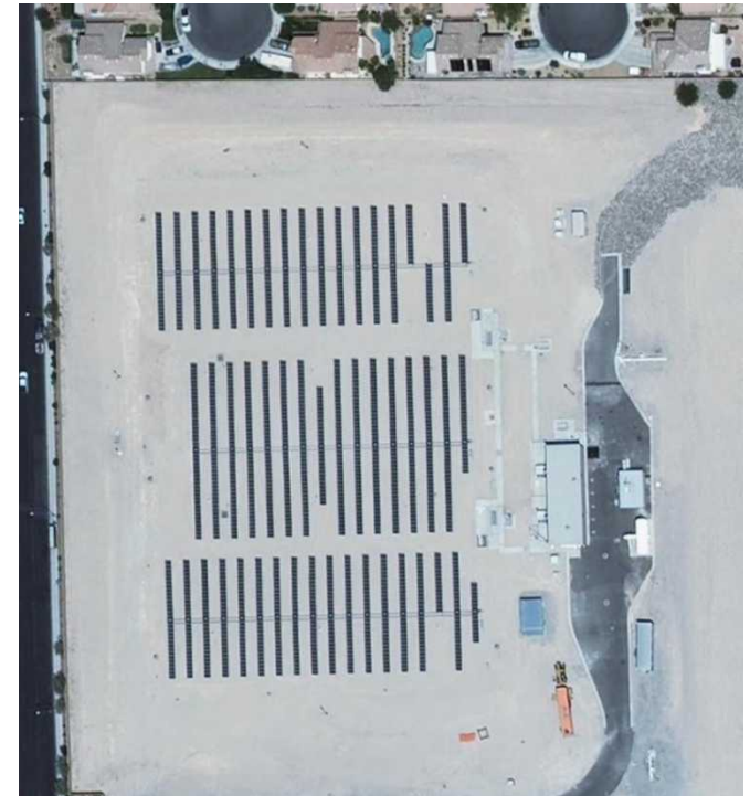
Ft Apache (353 kWp) Single Axis
