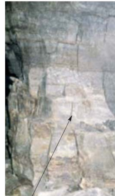
Fractured rock mass in rock pillar.
