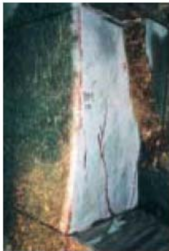
The fractures around the tunnel were a few centimetres deep.
