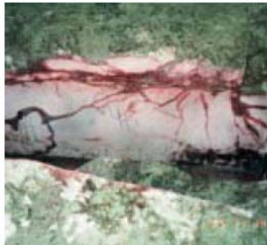
The fractures around a drilled-and-blasted tunnel are much deeper. They were around 30 centimetres in the walls.
