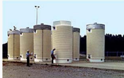
Spent fuel dry storage in casks Picture Courtesy: USNRC
