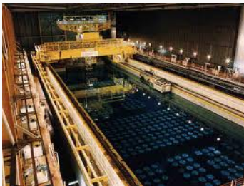
Onsite spent fuel pool ( wet storage ) Picture courtesy: http://world-nuclear.org
