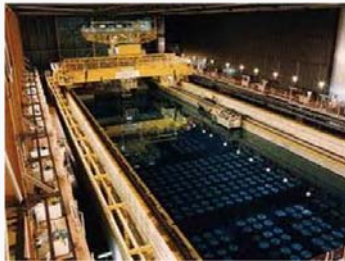
Onsite spent fuel pool (wet storage) Picture courtesy: http://world-nuclear.org
