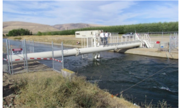
Instream Energy Systems turbine deployment at the Roza Canal site in Yakima, Washington.
