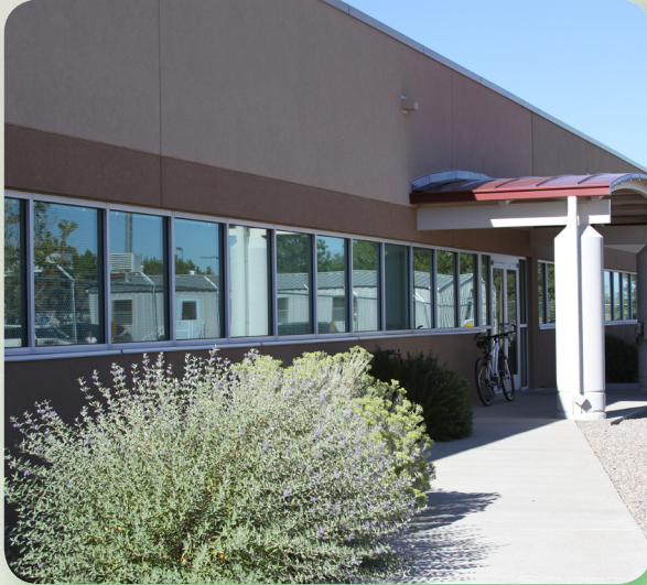
Building 750 – Reduced indoor water use 43%; reduced outdoor water use 79%; reduced annual energy consumption 25%.
