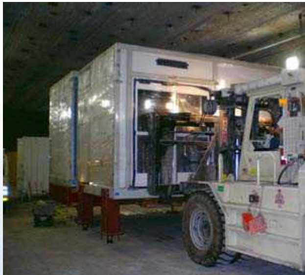
Enriched Xenon Observatory clean-room modules are put in place at WIPP.
