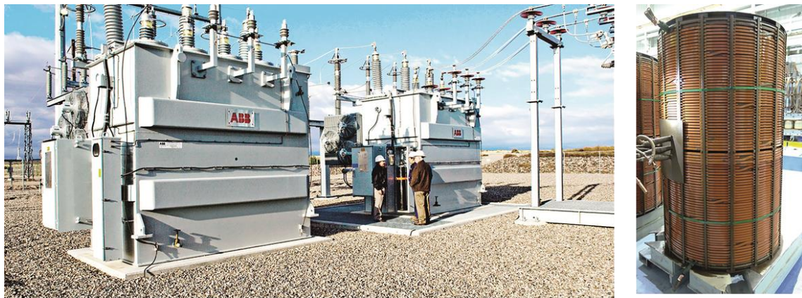
Figure 3-1. Image of ABB commercial grid scale transformers and a representative helical transformer winding, utilizing copper conductors and Kraft paper insulation.
