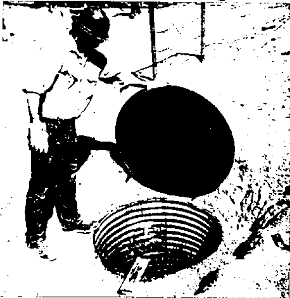
VIEW OF CORRUGATED PIPE WITH THE 1/2" STEEL LID OPEN
