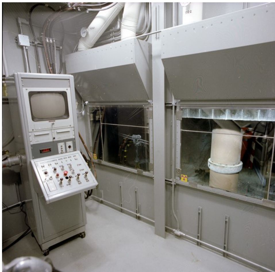
Figure 19. View of Z-9 Crib Mining Operations Cubicle and Windows into Z-9 (image 72698-30CN from Hanford Site photo archive)
