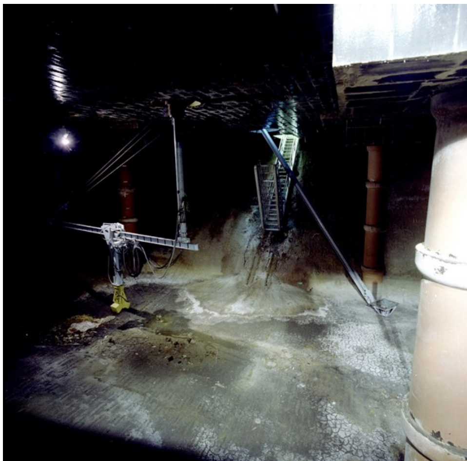
Figure 18. Interior View of Z-9 Crib and Crib Soil Removal Equipment Prior to Mining Operations (taken through operations cubicle window; image 72698-32CN from Hanford Site photo archive)
