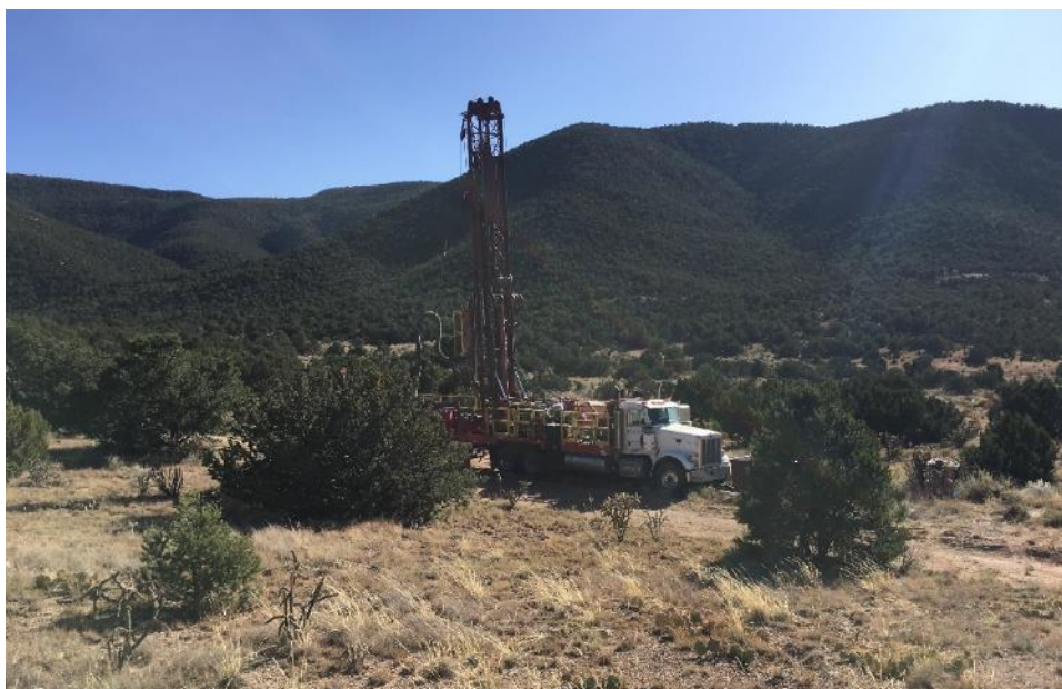
Groundwater monitoring well installation in Lurance Canyon
