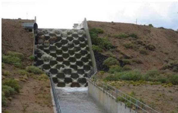
“Dragon’s teeth,” stormwater energy dissipater located south of SWSP-05.
