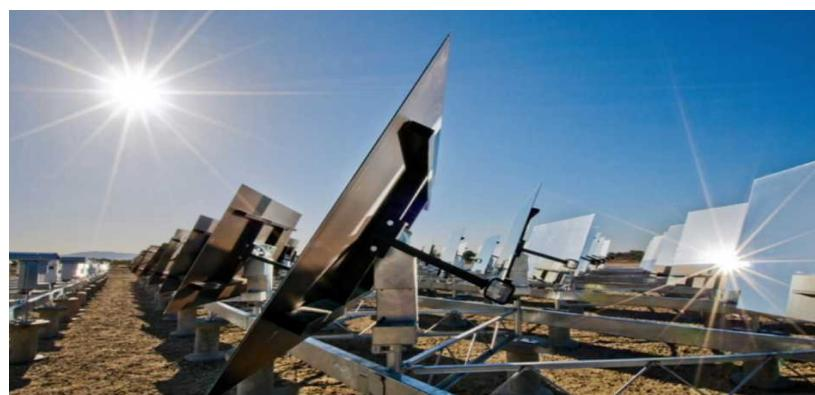
*Key to eSolar's technology is precise, automated calibration and control of thousands of their mass-produced sun-tracking heliostats, or solar reflectors.*
