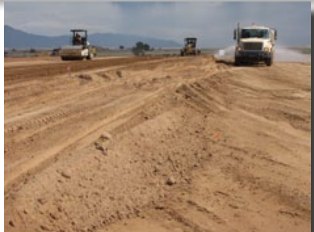
Construction of the Native Soil Layer, Lift #6. 7/14/09
