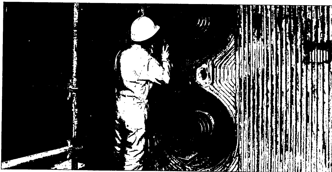
Figure 4-6 An original cell burner as seen from the burner. Each cell is comprised of two closely-spaced circular burners as shown in this photo. Vertical centerline spacing between each burner is approximately 4.5 feet.
