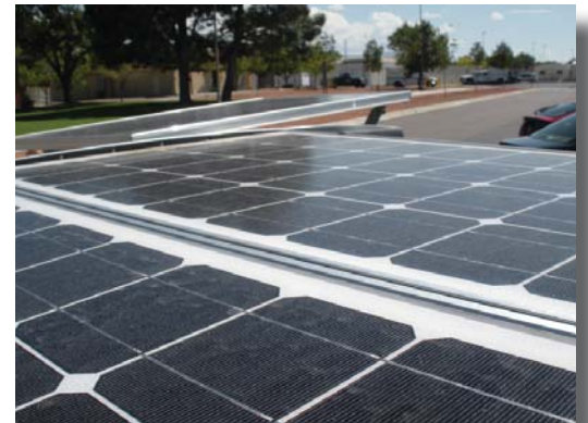
Polycrystalline panels collect solar energy that is sent to the batteries.
