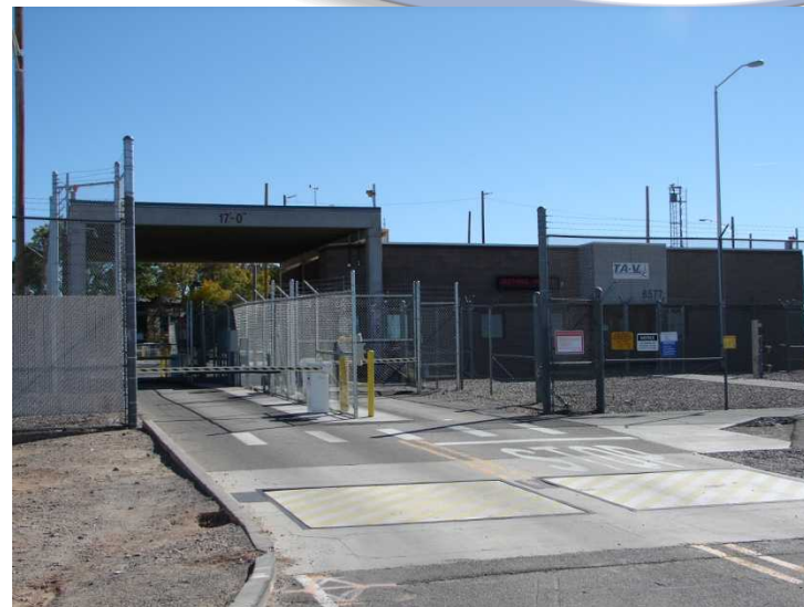
Entry Control Portal (ECP)
