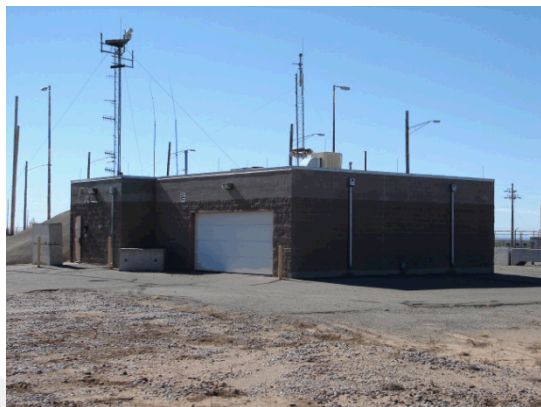
Central Alarm Station (CAS)
