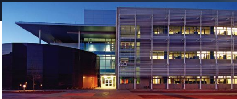
Sandia MESA Facility
