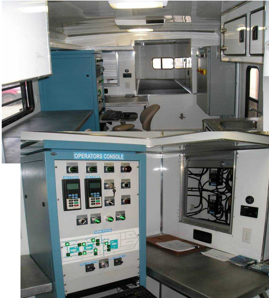
View of Controls: Operator Console, Motor Control and DAS Panel
