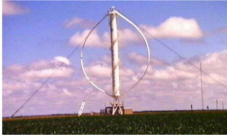
500kW 34m VAWT Test Bed
