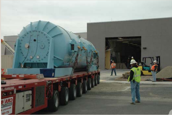
An accelerator weighing more than 100,000 pounds is moved into the IBL Tandem Vault from Building 884.
