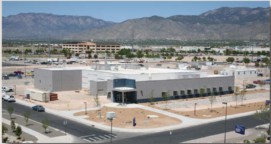
The Ion Beam Laboratory at the intersection of K and 18th Streets.
