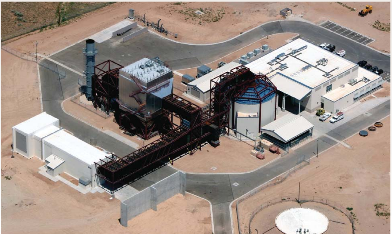
Thermal Test Complex as built by the Hensel Phelps Construction Company.
