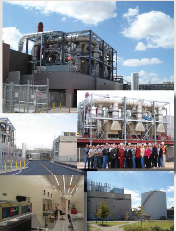
Clockwise, top to bottom, MicroFab exhaust system, project team, Central Utility Building, new cleanroom, service road and pipe bridge.
