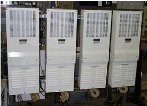
Example for 4 parallel inverters
