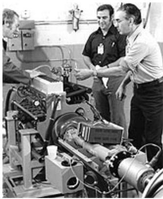
Bill Kent, Denny Spanger, and Harvey Pouliot discuss the Pouliot variable displacement engine.
