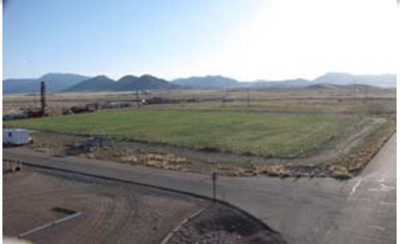
CWL At-Grade Vegetative Soil Cover in April 2010
