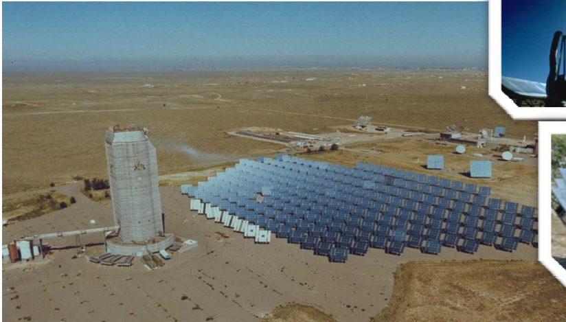
Solar-thermal Generation at Sandia's NSTTF
