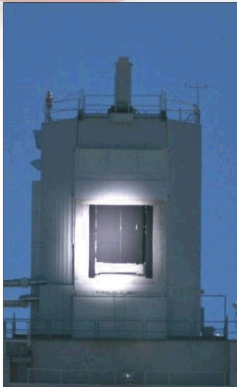
CAVITY MOLTEN SALT RECEIVER
