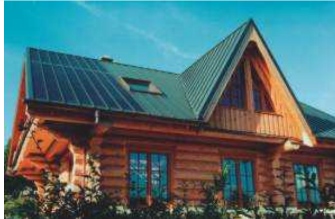
3kW a-Si rooftop at Sandia's Distributed Energy Technologies Laboratory (DETL)
