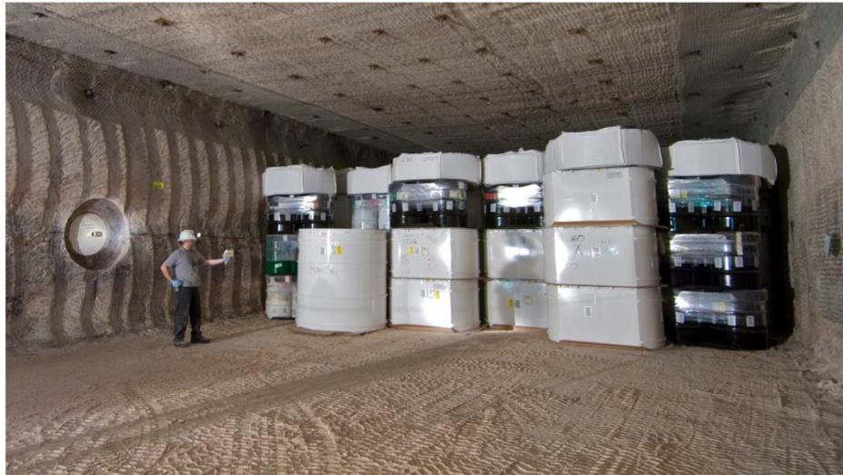
**Contact Handled (CH) Waste is emplaced in rooms mined out of ancient saltbeds.**
