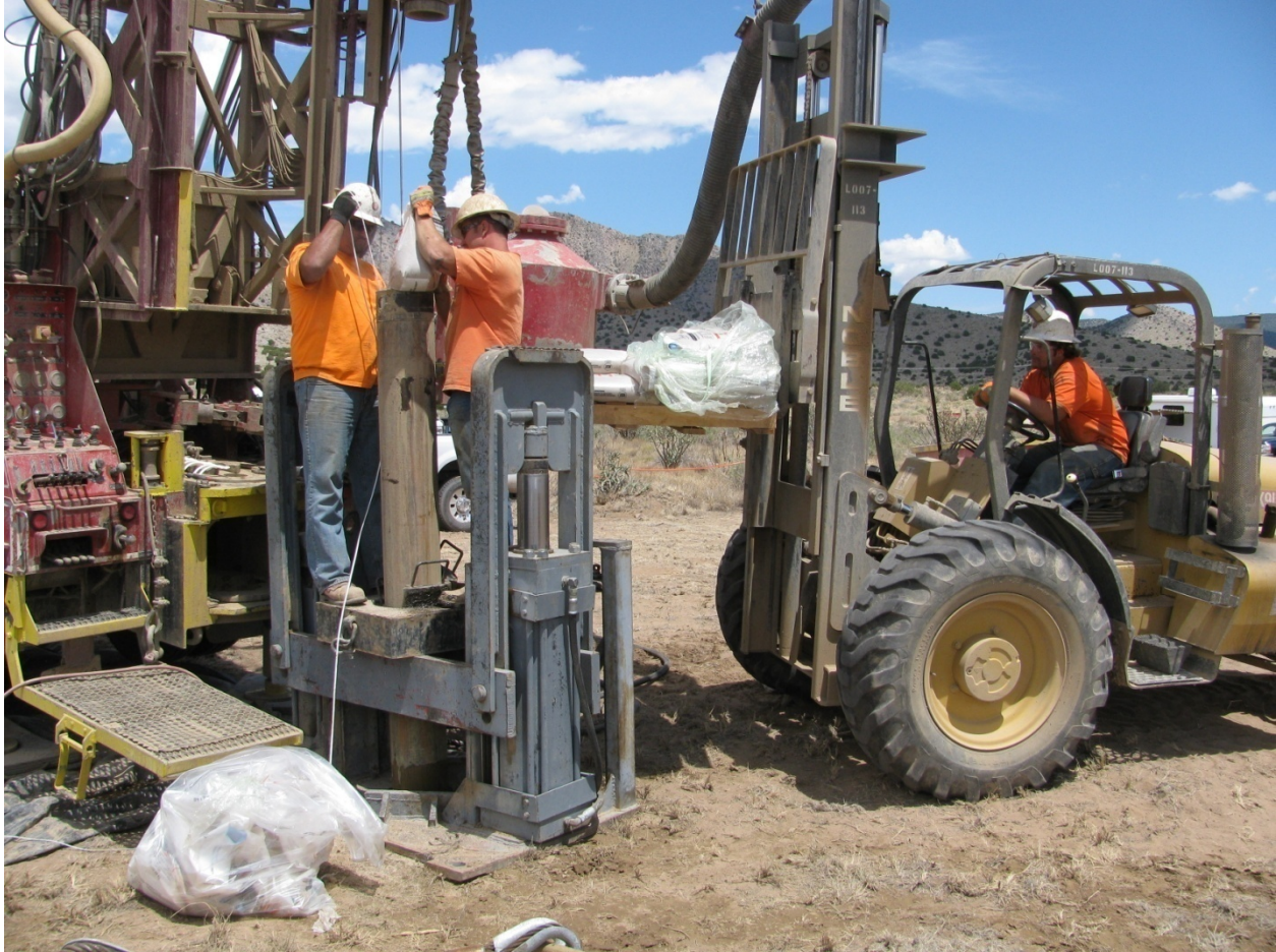
Figure 2-2 Installing the sand pack for monitoring well CCBA-MW1 at SWMU 8. View to the northeast, August 13, 2011.
