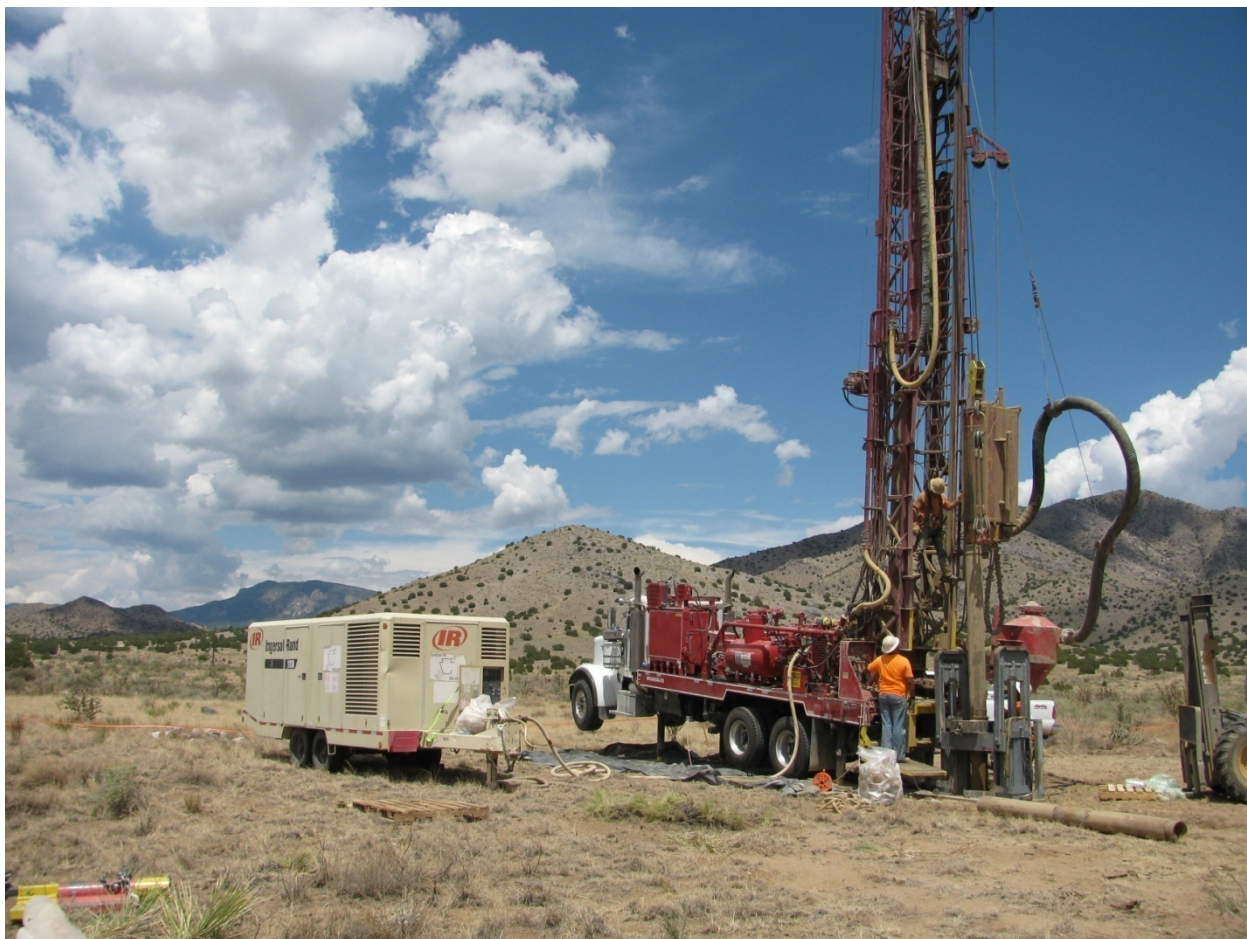
Figure 2-1 Pulling the drive casing while installing well materials at monitoring well CCBA-MW1, located at the southwestern corner of SWMU 8. View to the northeast, August 13, 2011.
